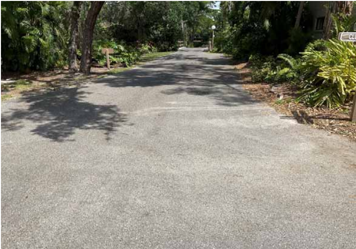
Paving - Brookhouse Drive
