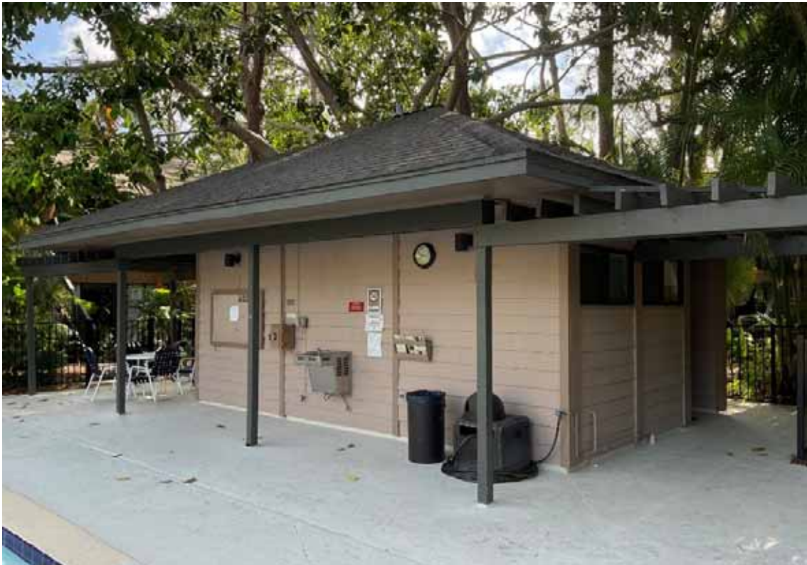
Glenhouse Pool Bldg
