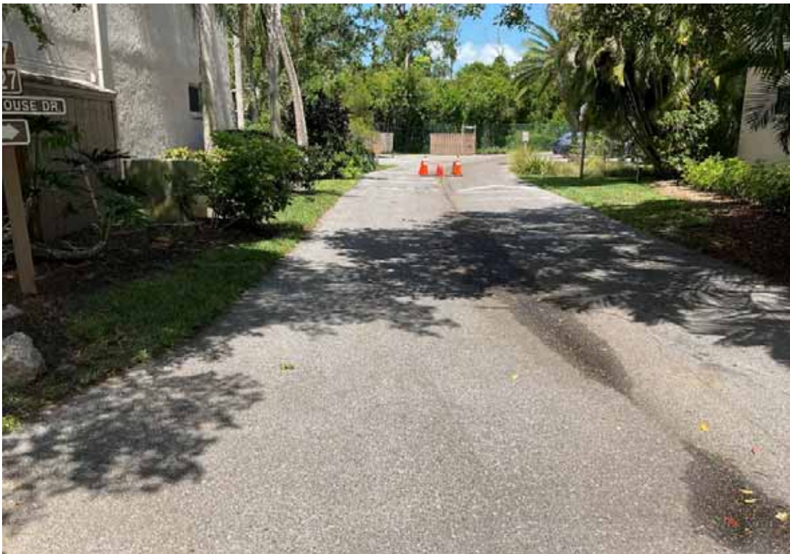
Paving - Brookhouse Drive
