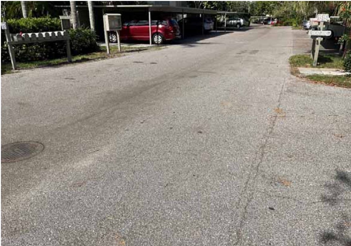
Paving - Pelican Point Drive
