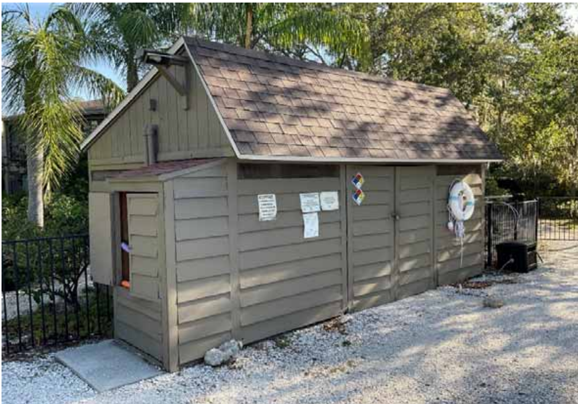
Pavilion Pool Equipment Bldg
