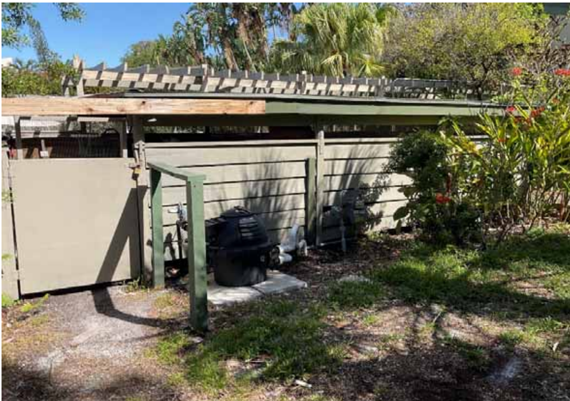
Wilbanks Pool Equipment Bldg
