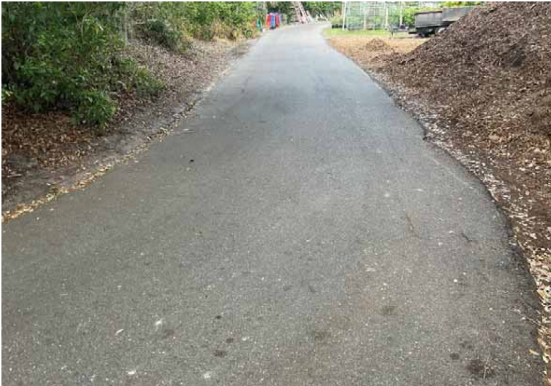
Paving - Maintenance Yard Driveway
