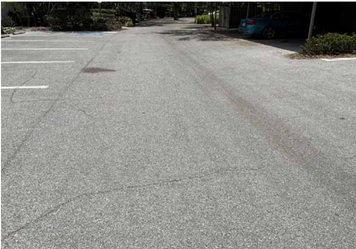
Paving - Boathouse Circle
