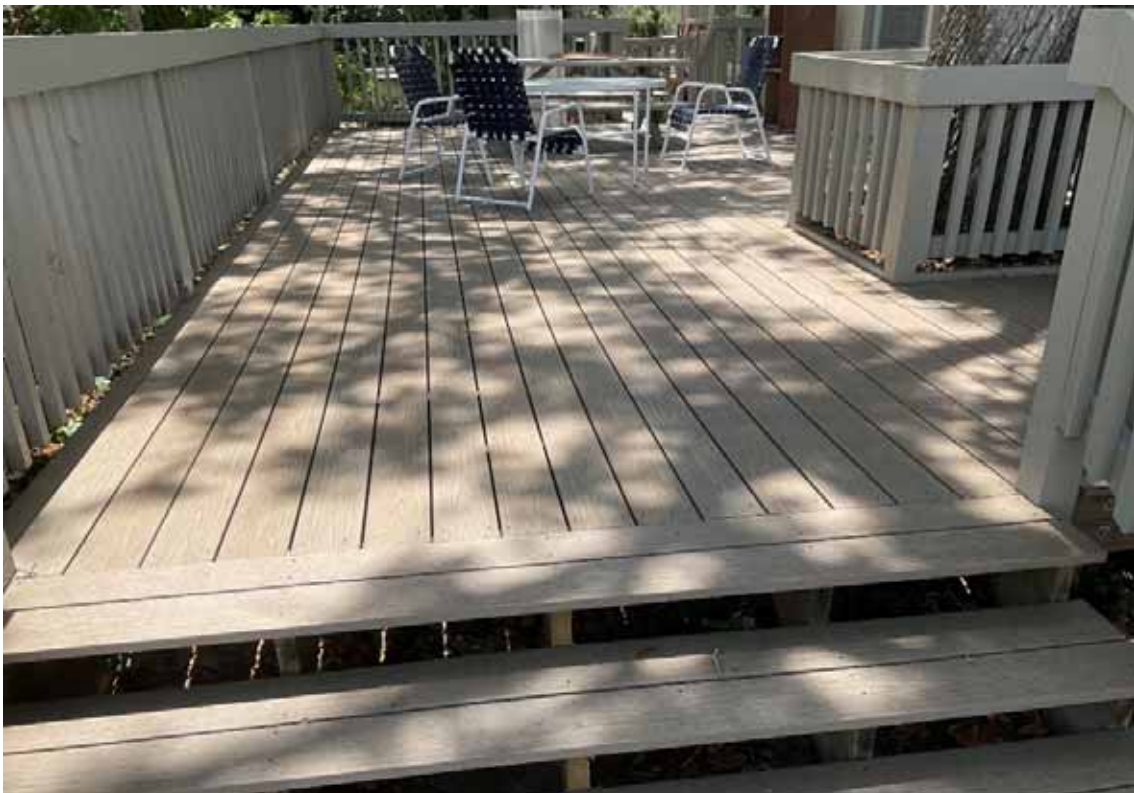
Harbor Club Deck - Rear
