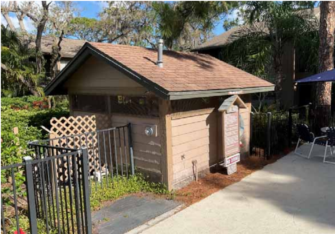
Glenhouse Pool Equipment Bldg
