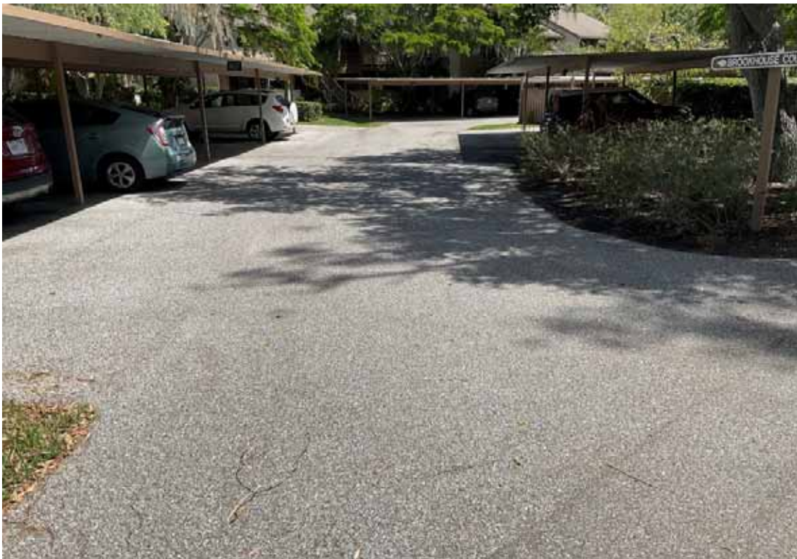
Paving - Brookhouse Court
