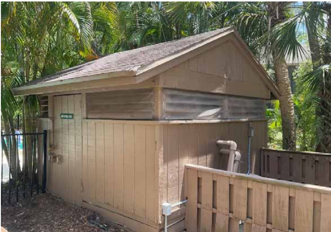
Brookhouse Pool Equipment Bldg
