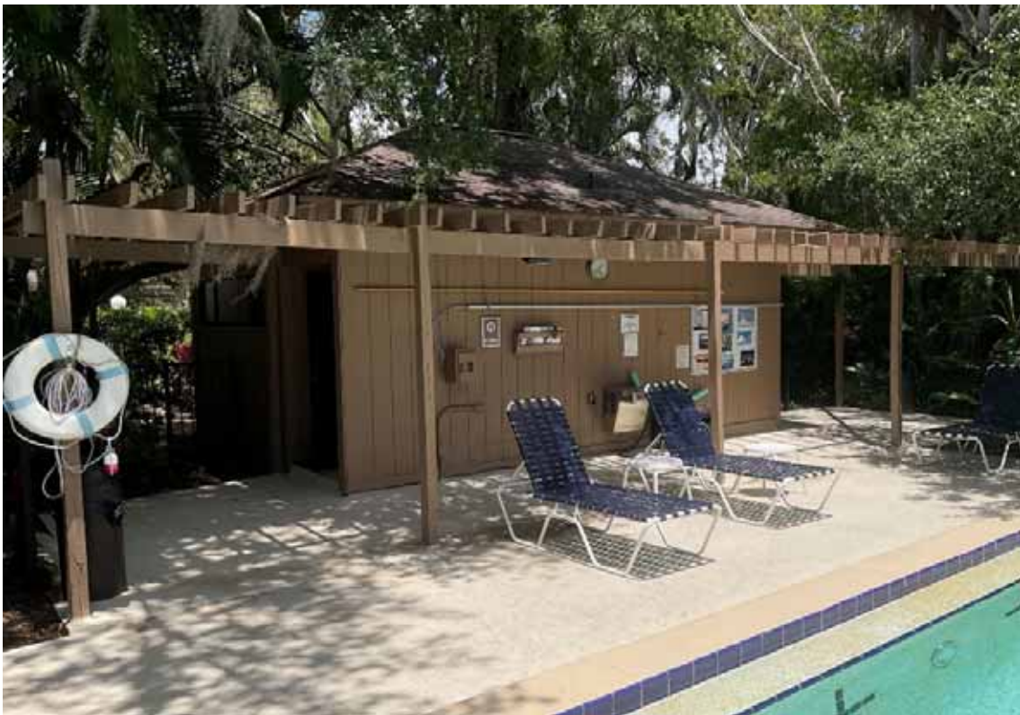
Brookhouse Pool Bldg
