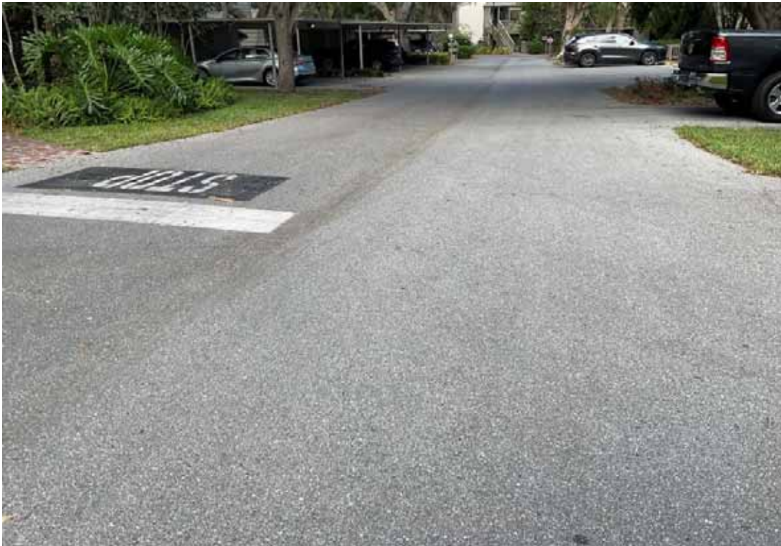
Paving - Bayhouse Court
