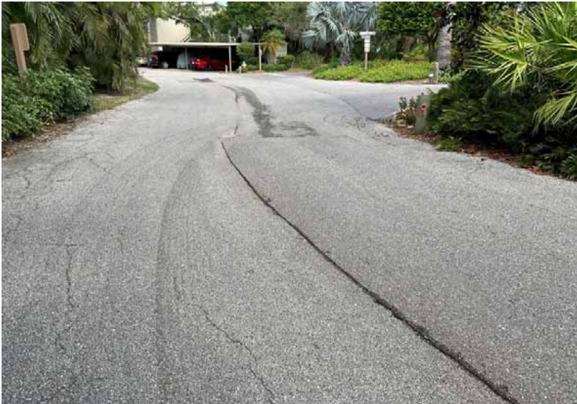
Paving - Bayhouse Point Drive
