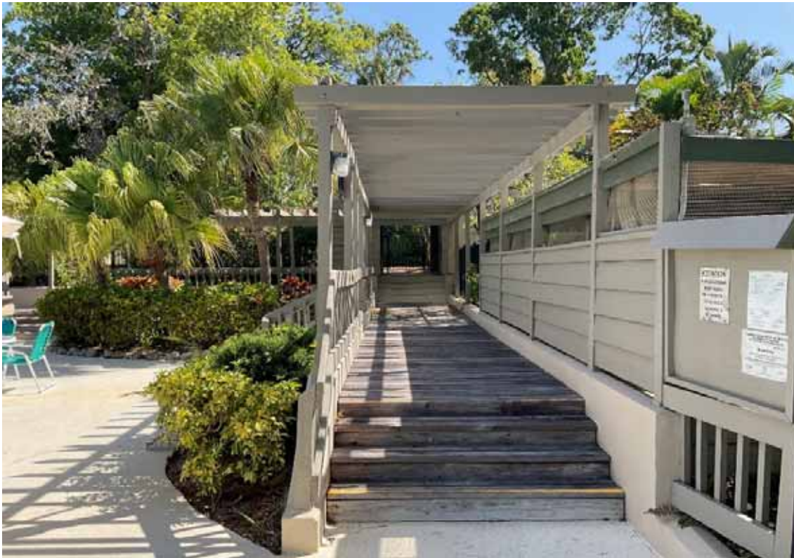
Wilbanks Pool Trellis
