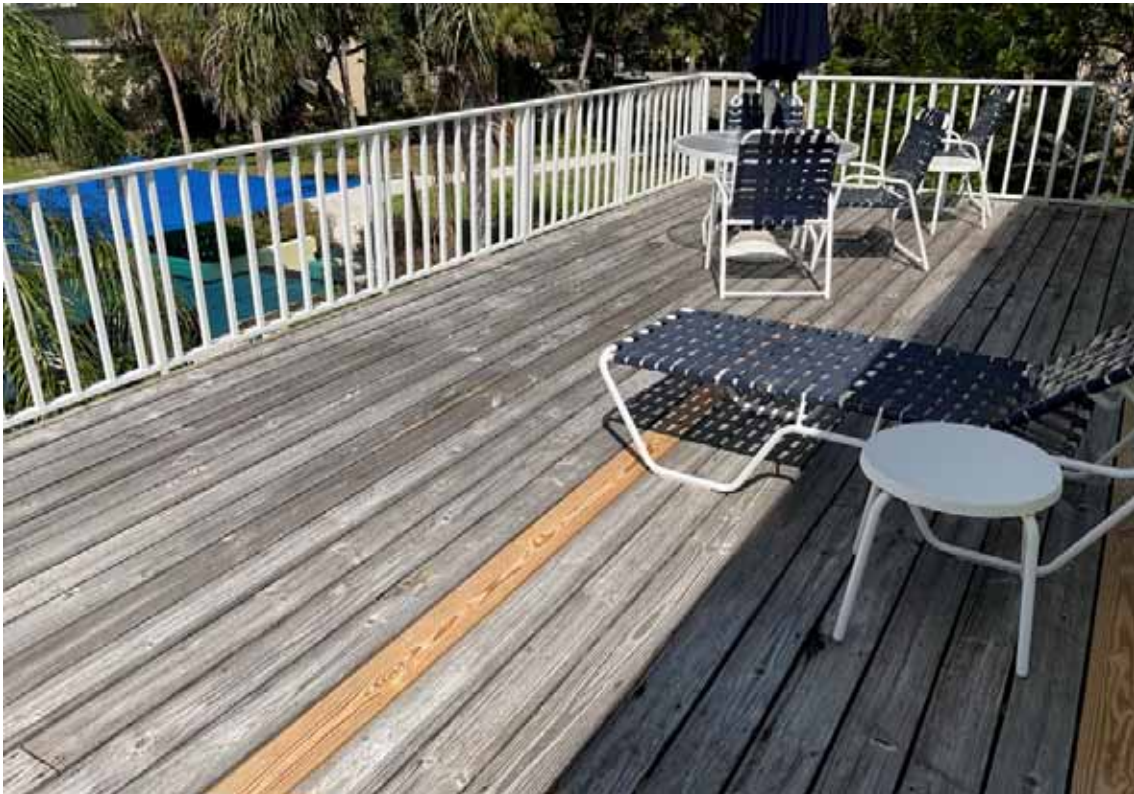
Wilbanks Bldg Second Floor Deck
