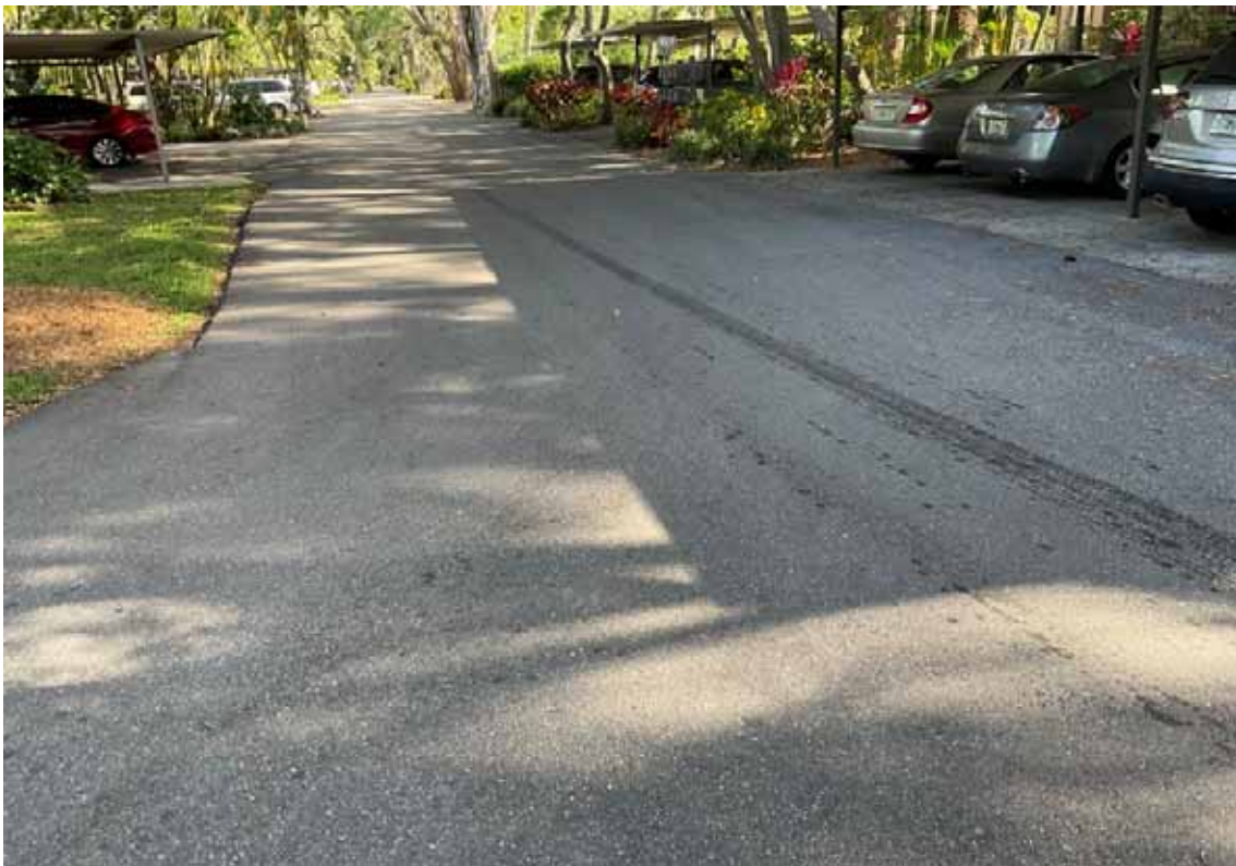
Paving - Bayhouse Point Drive
