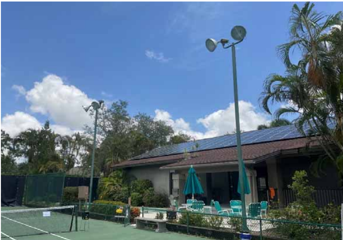
Pavilion Tennis Court Lighting
