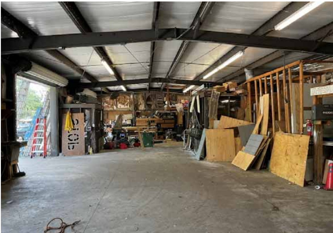
Maintenance Bldg Shop
