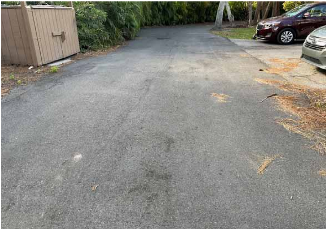
Paving - Glenhouse Drive
