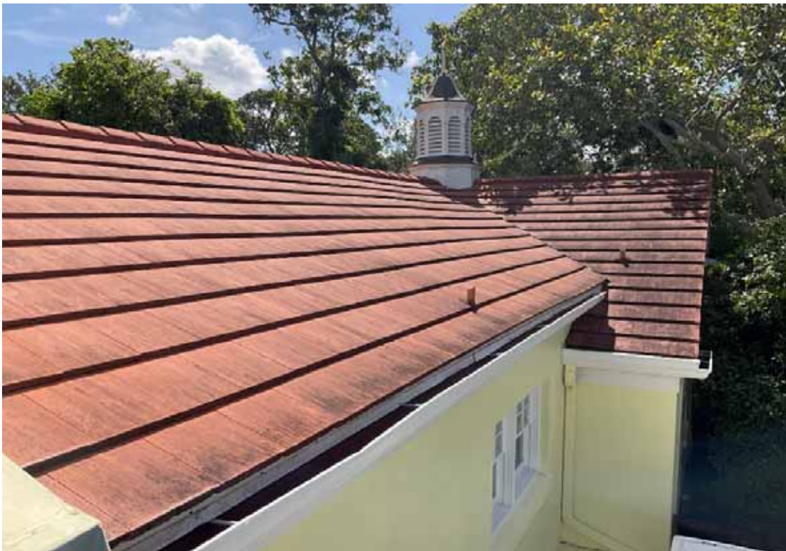
Wilbanks Bldg Roof
