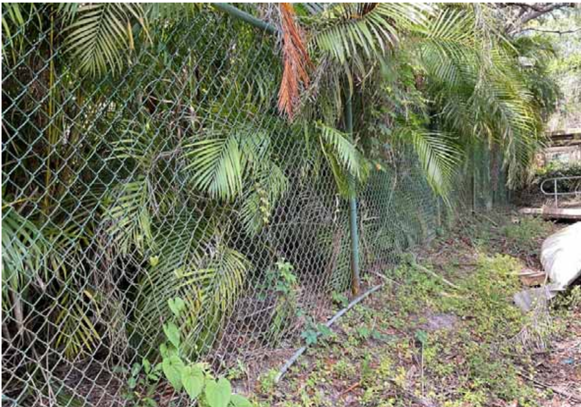
Fence - Maintenance Yard
