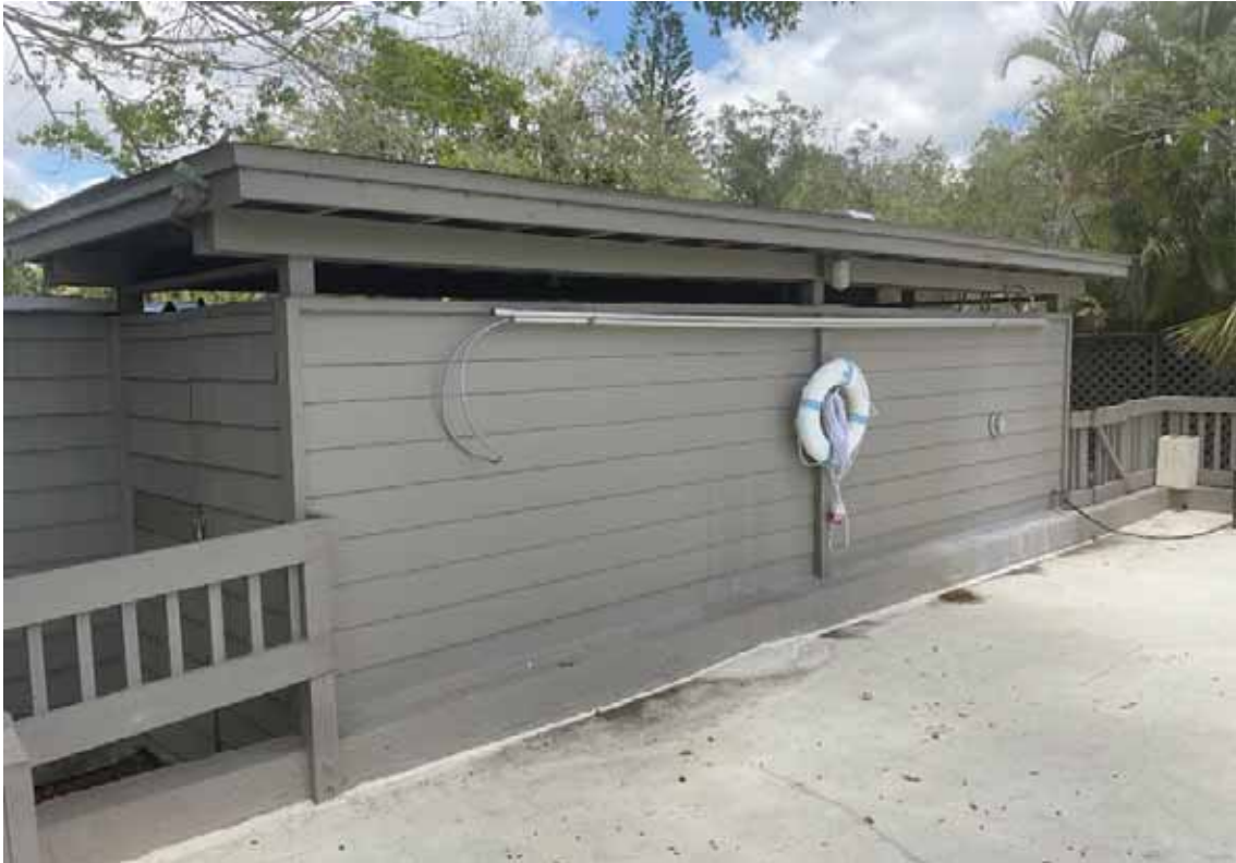
Far Harbor Pool Equipment Bldg
