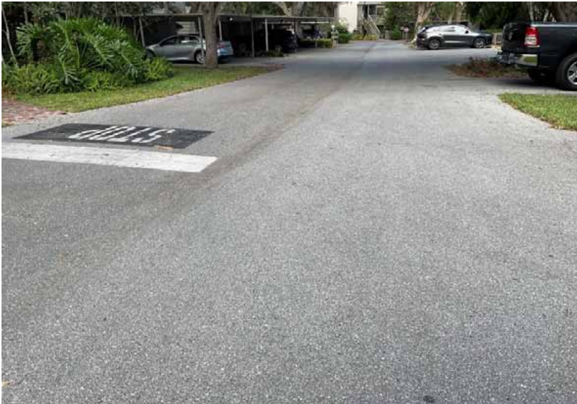
Paving - Bayhouse Court
