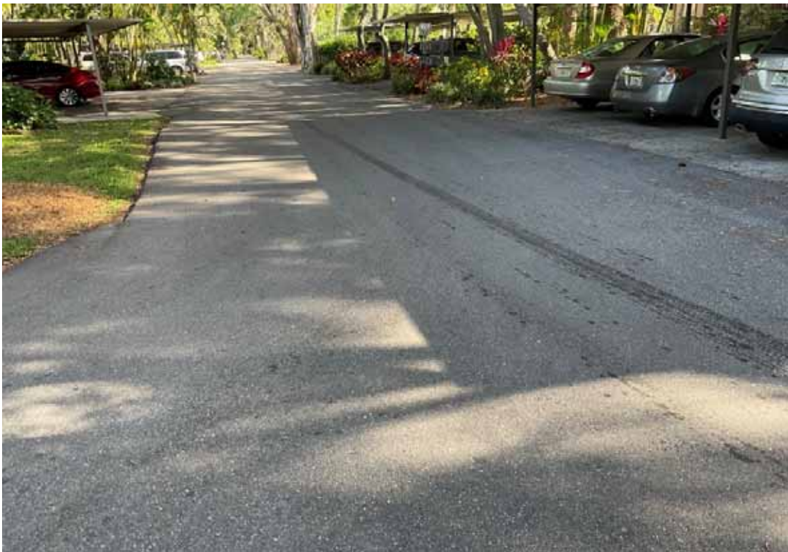
Paving - Bayhouse Point Drive
