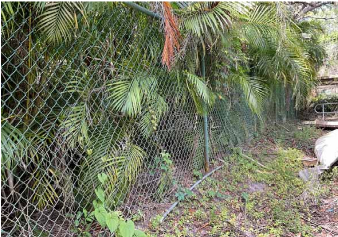
Fence - Maintenance Yard
