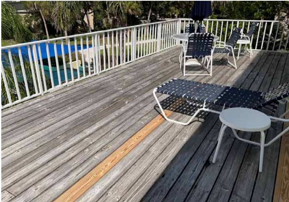
Wilbanks Bldg Second Floor Deck
