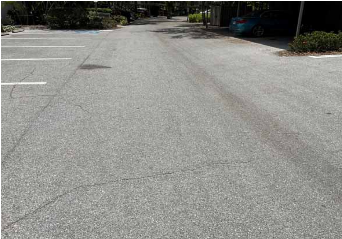
Paving - Boathouse Circle
