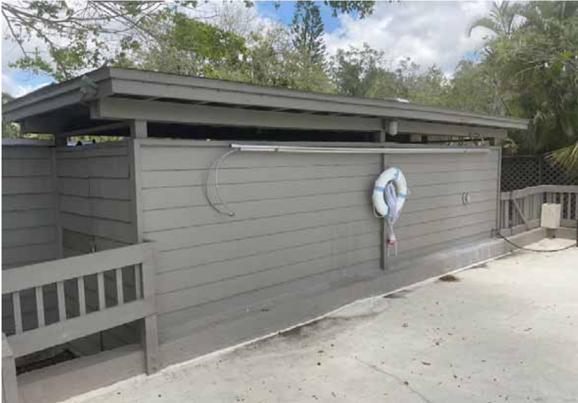
Far Harbor Pool Equipment Bldg
