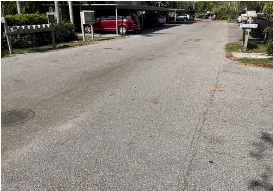
Paving - Pelican Point Drive
