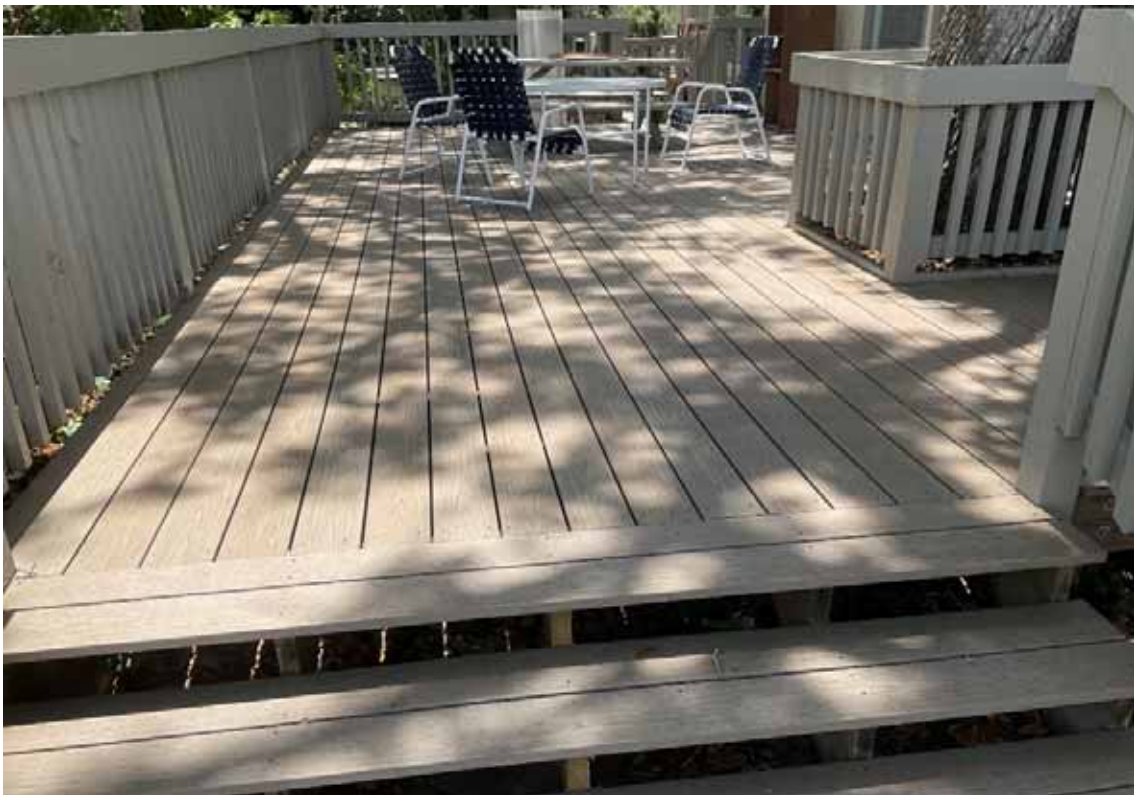
Harbor Club Deck - Rear
