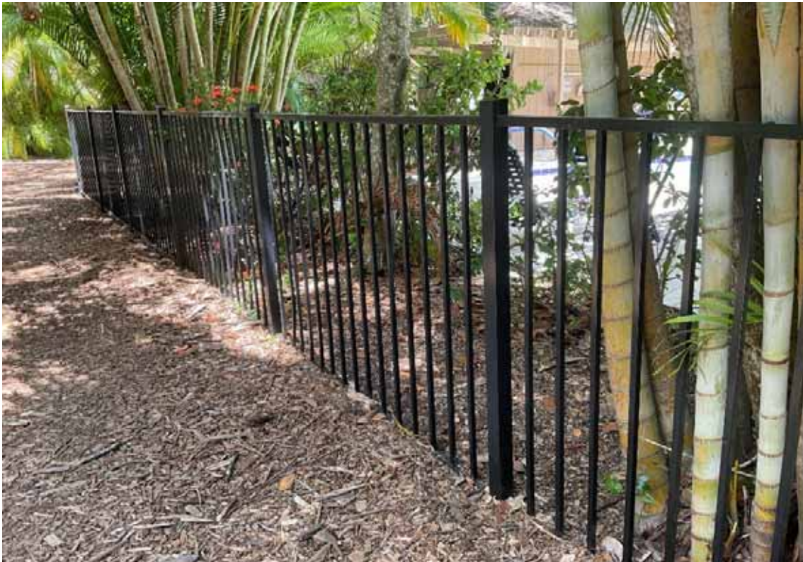
Brookhouse Pool Fence
