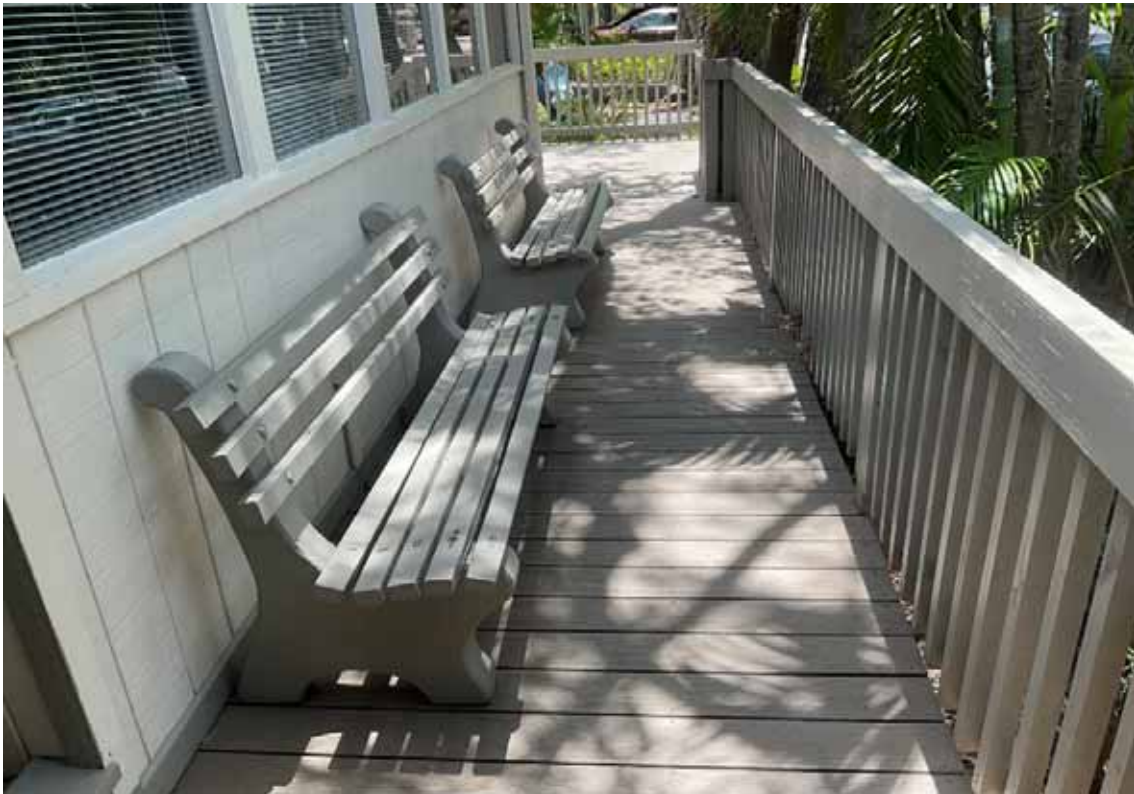
Harbor Club Deck - Front
