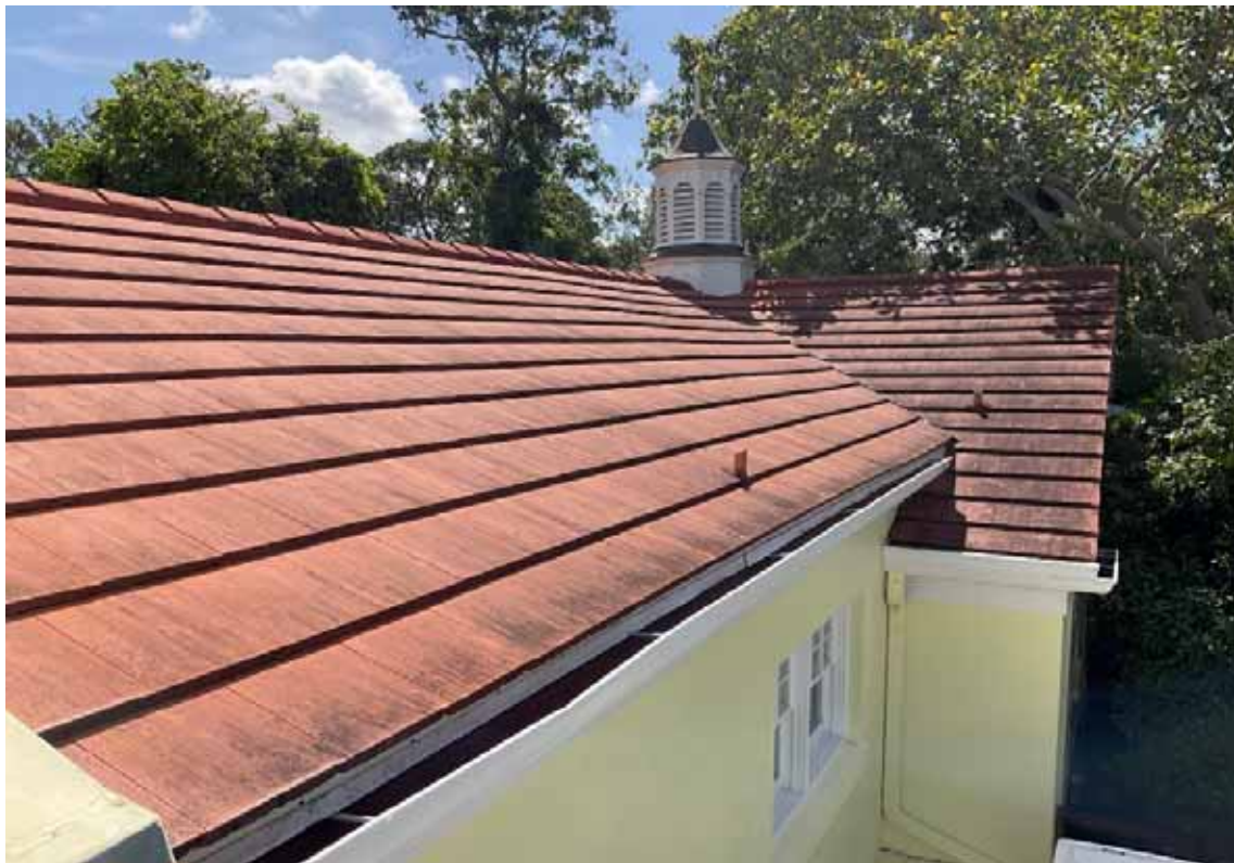
Wilbanks Bldg Roof
