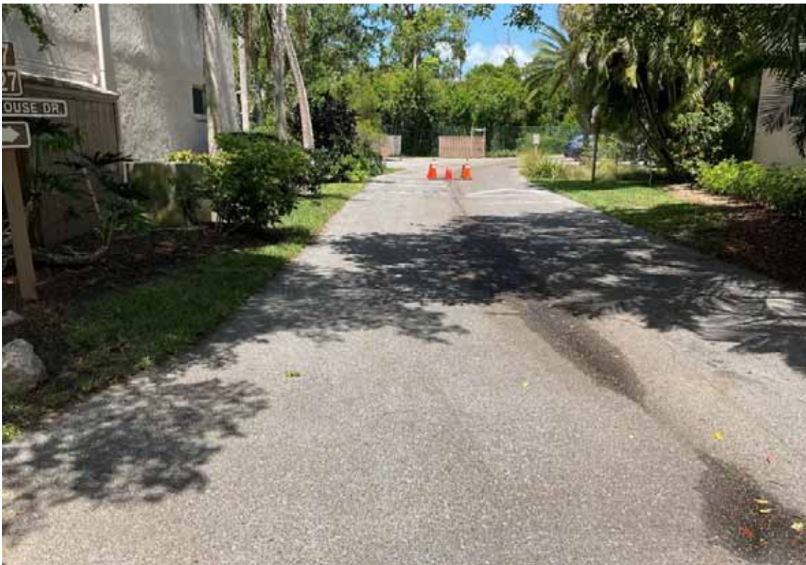
Paving - Brookhouse Drive
