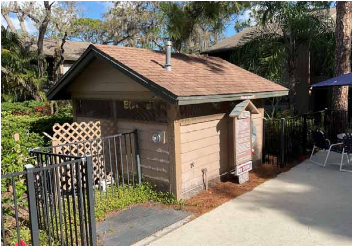
Glenhouse Pool Equipment Bldg
