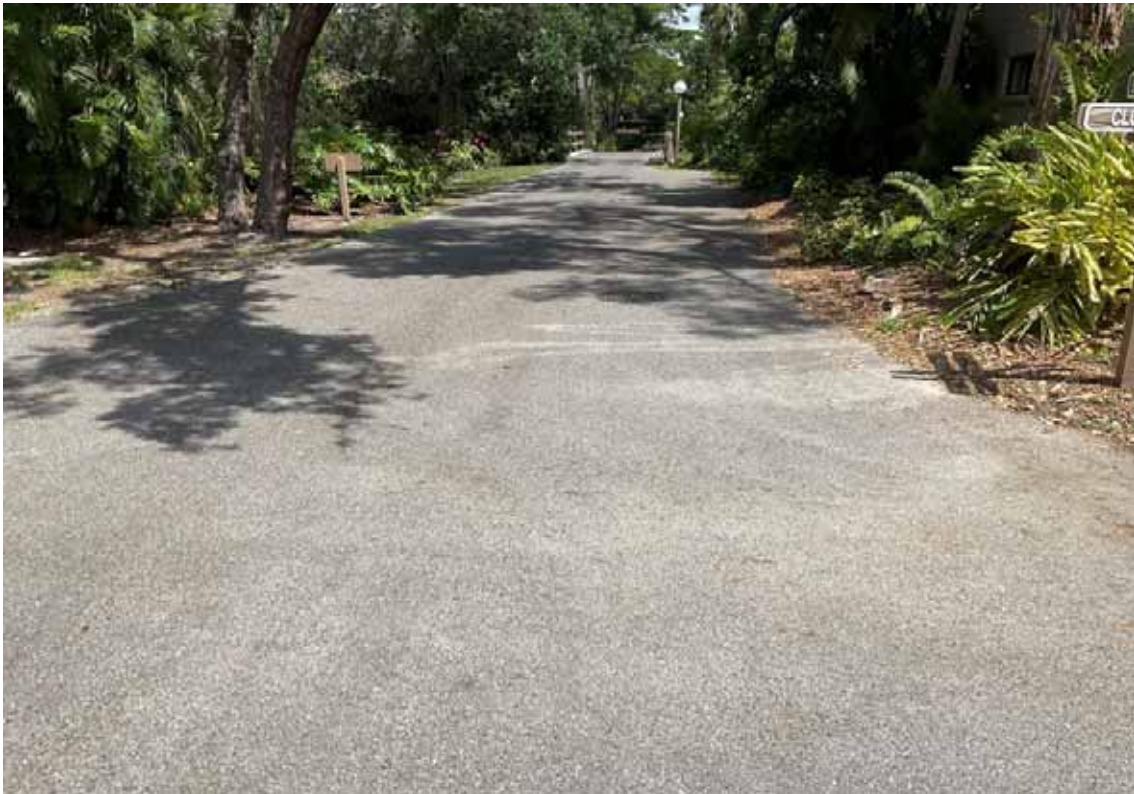
Paving - Brookhouse Drive
