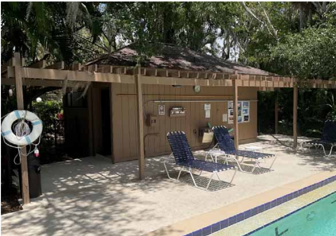
Brookhouse Pool Bldg
