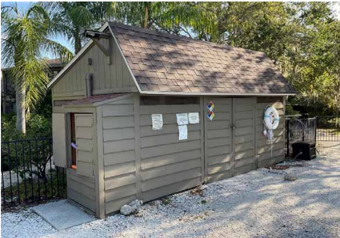
Pavilion Pool Equipment Bldg
