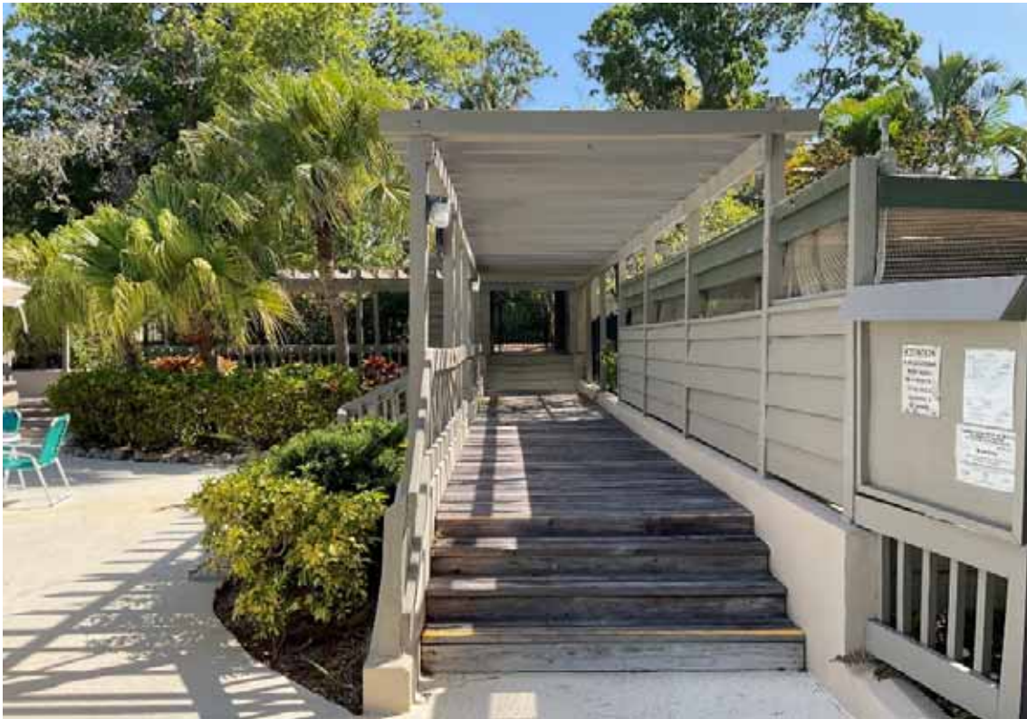
Wilbanks Pool Trellis
