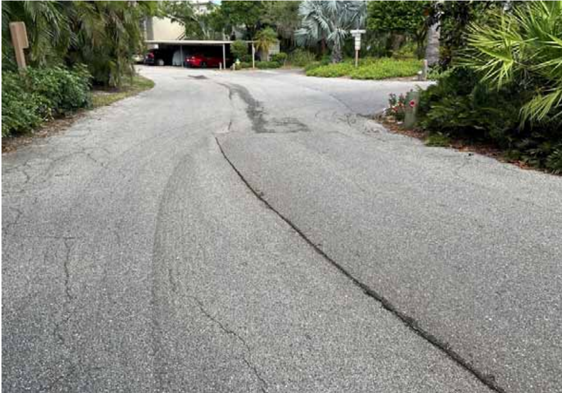
Paving - Bayhouse Point Drive
