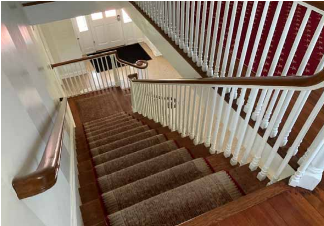
Wilbanks Bldg Stairway
