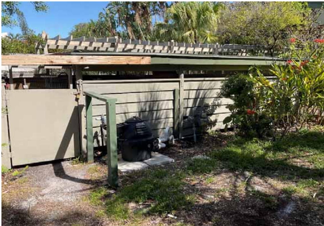
Wilbanks Pool Equipment Bldg
