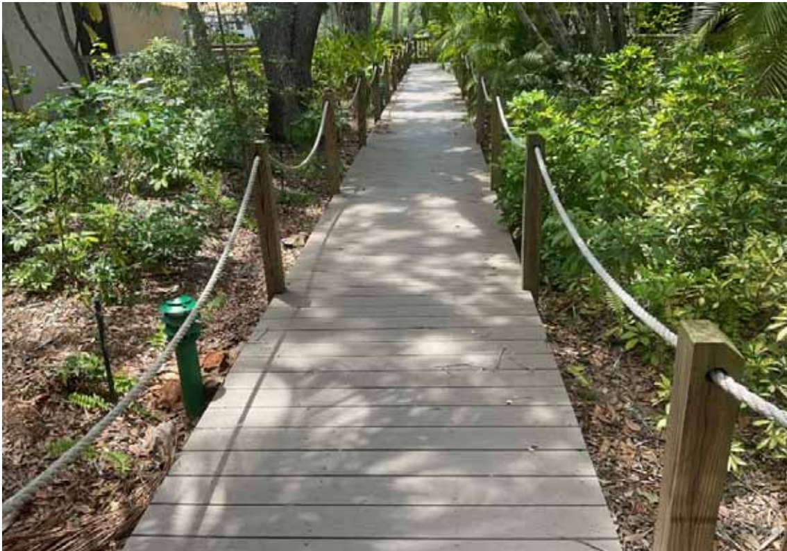
Harbor Marina Boardwalk
