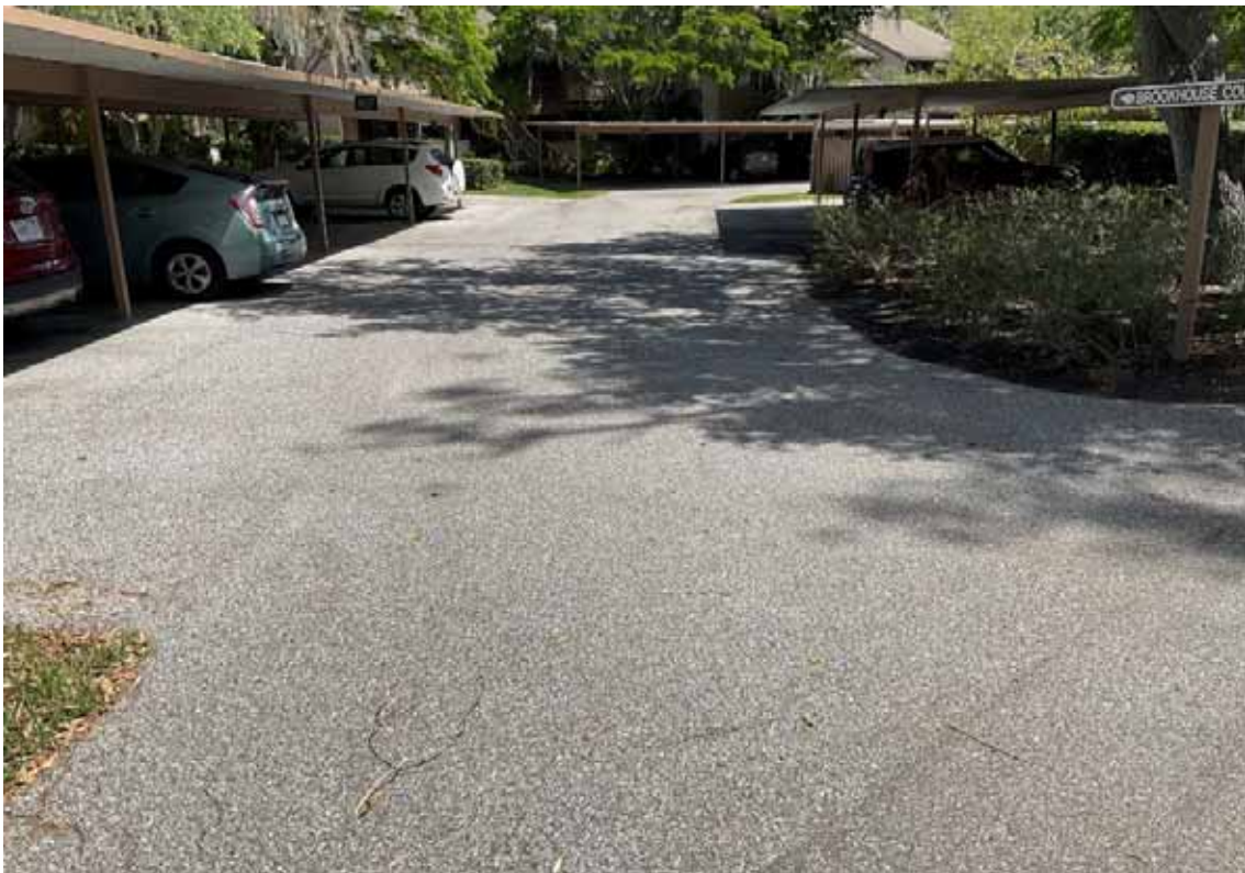
Paving - Brookhouse Court
