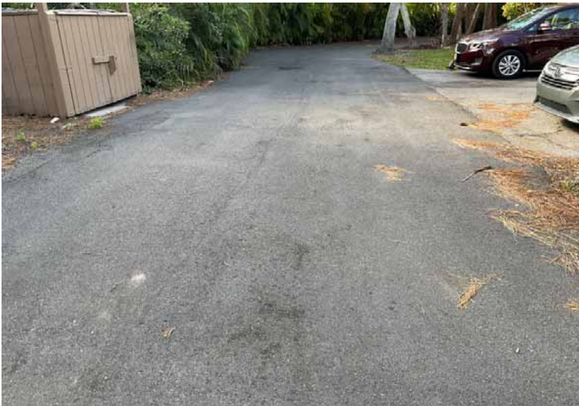
Paving - Glenhouse Drive
