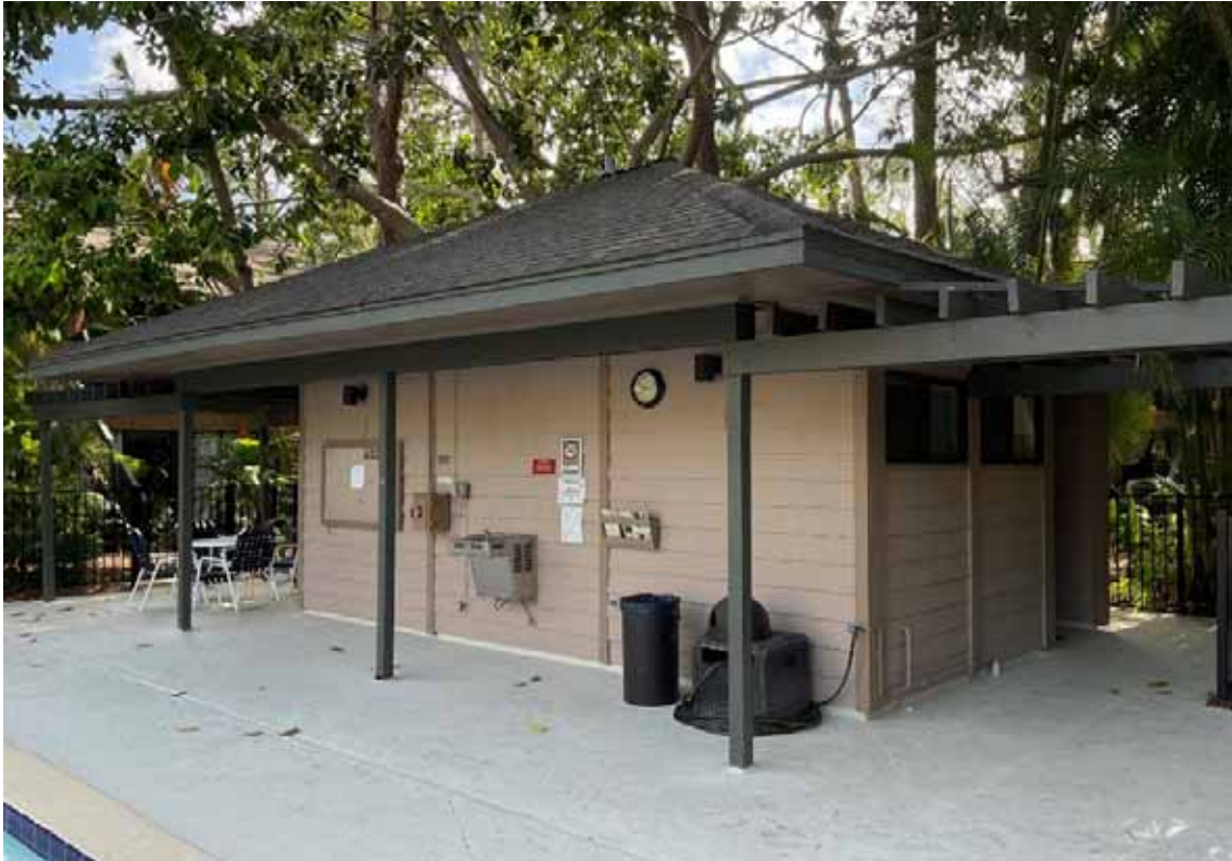
Glenhouse Pool Bldg
