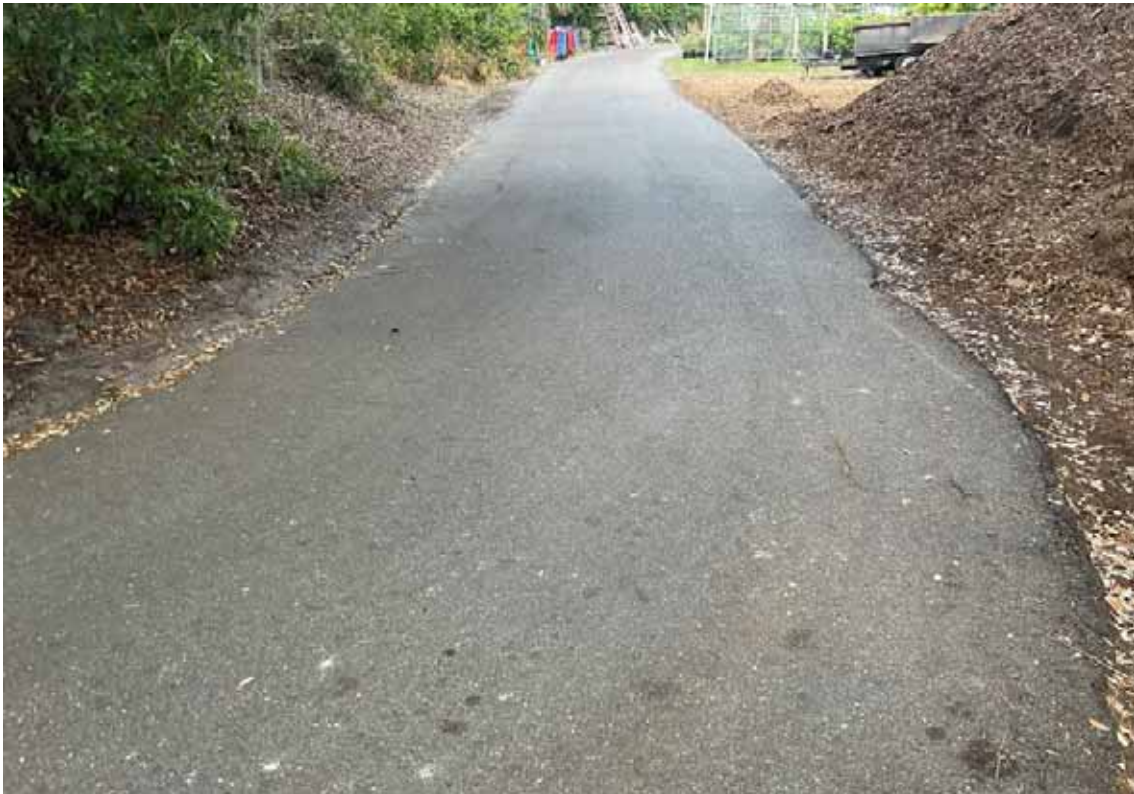
Paving - Maintenance Yard Driveway
