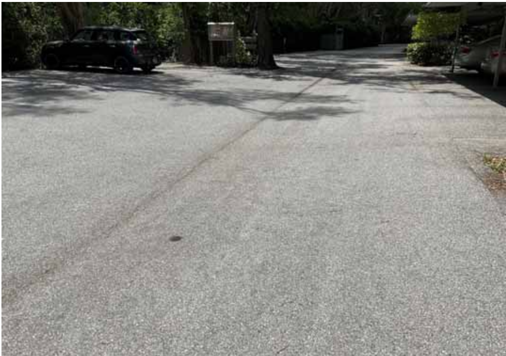
Paving - Clower Creek Drive
