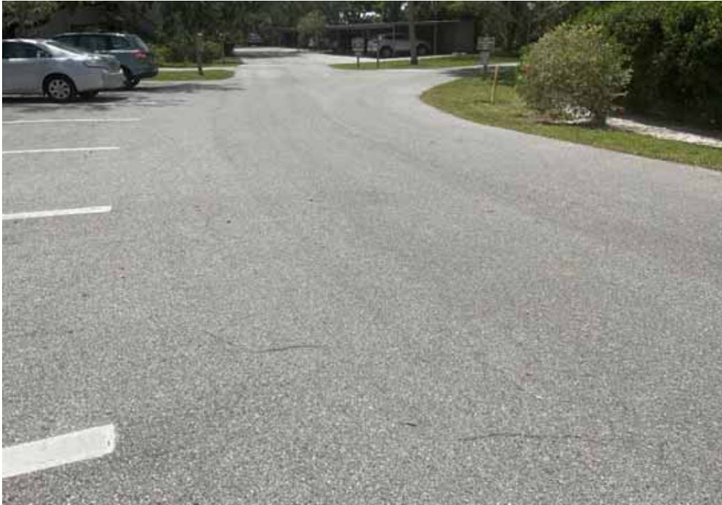
Paving - Clower Creek Drive
