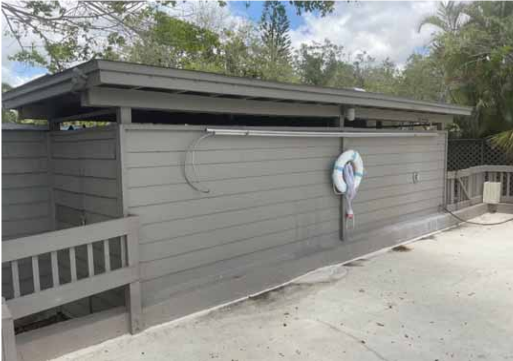
Far Harbor Pool Equipment Bldg
