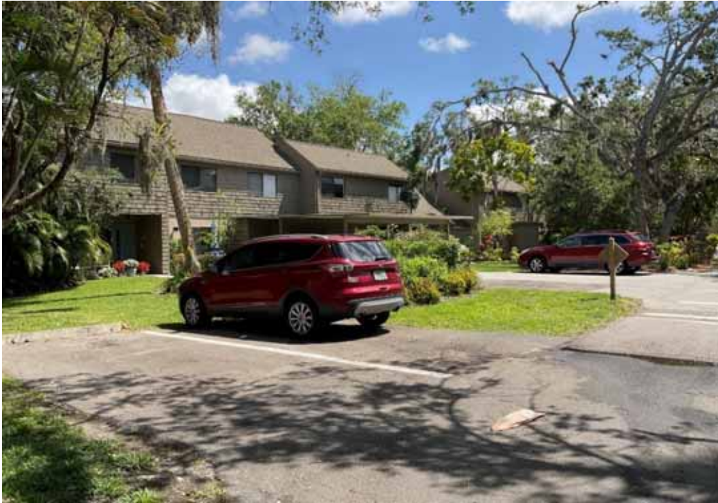
Treehouse Condo Bldg - 6 Unit
