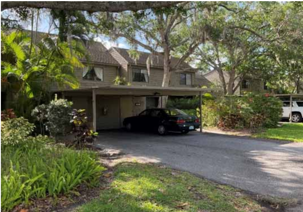
Treehouse Condo Bldg - 6 Unit
