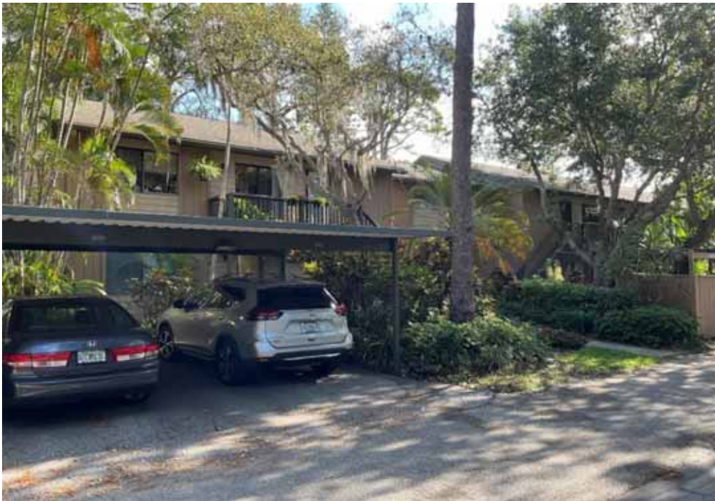
Glenhouse Condo Bldg - 8 Unit
