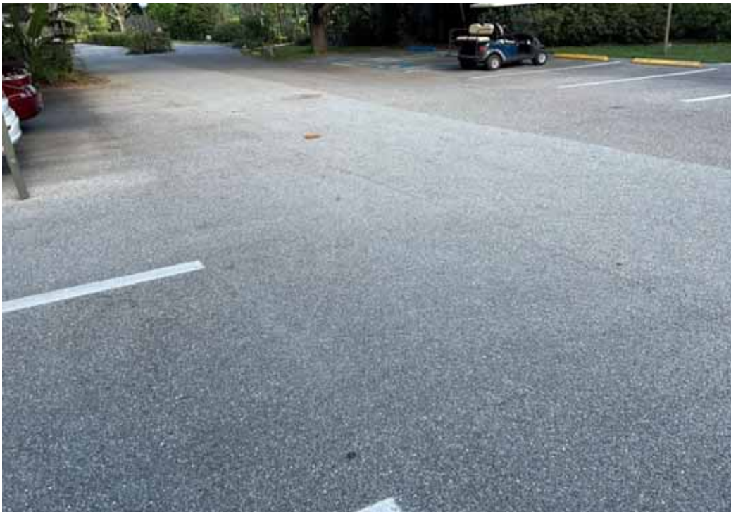
Paving - Pelican Cove Road
