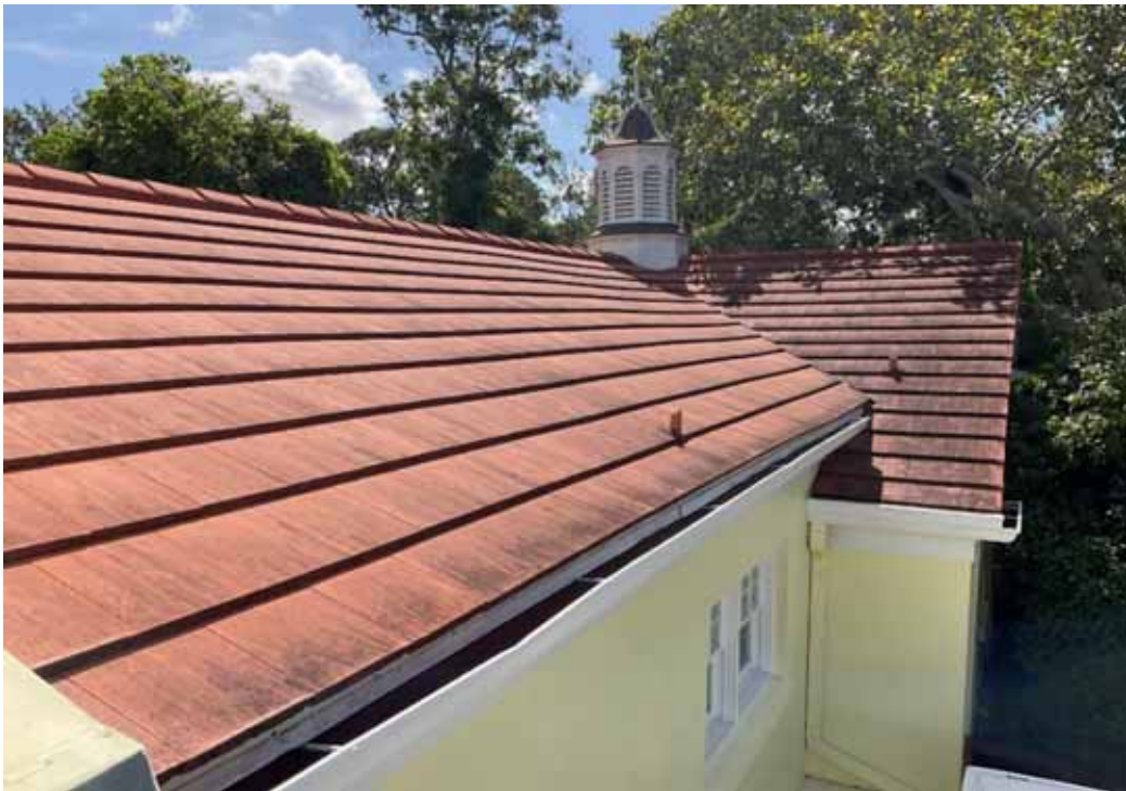
Wilbanks Bldg Roof
