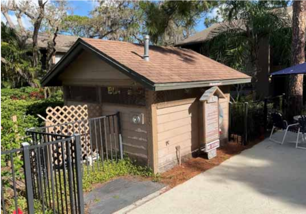
Glenhouse Pool Equipment Bldg
