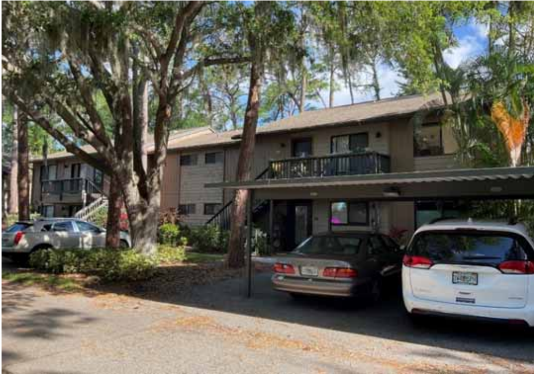
Glenhouse Condo Bldg - 4 Unit
