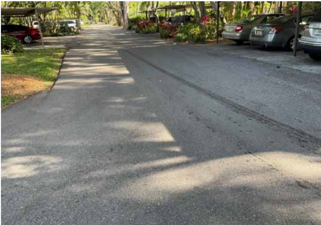
Paving - Bayhouse Point Drive
