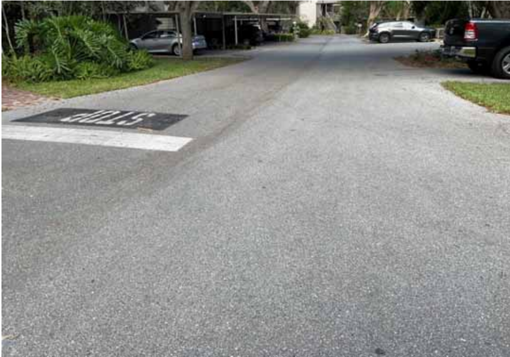
Paving - Bayhouse Court
