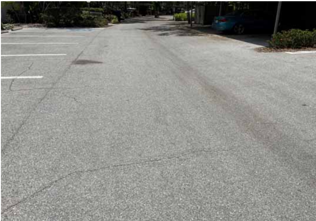
Paving - Boathouse Circle
