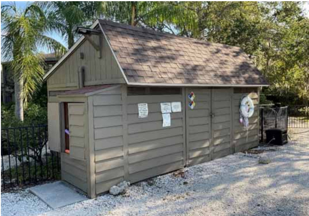
Pavilion Pool Equipment Bldg
