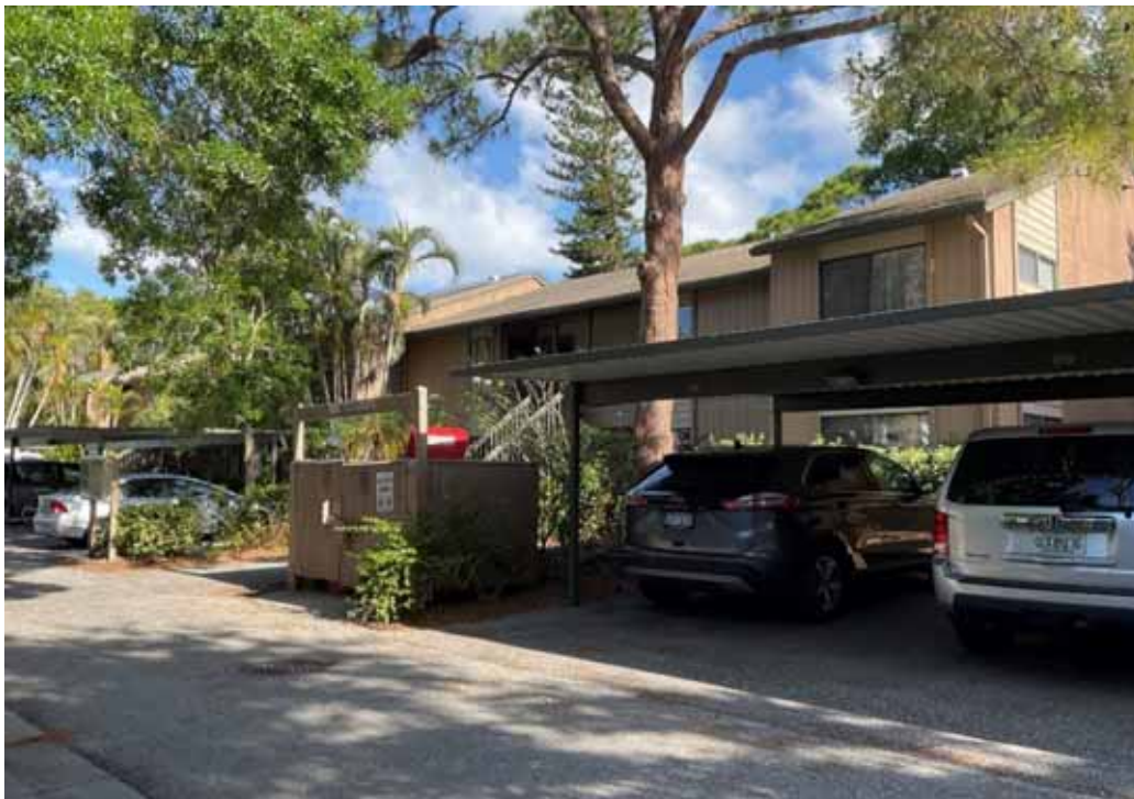
Glenhouse Condo Bldg - 8 Unit
