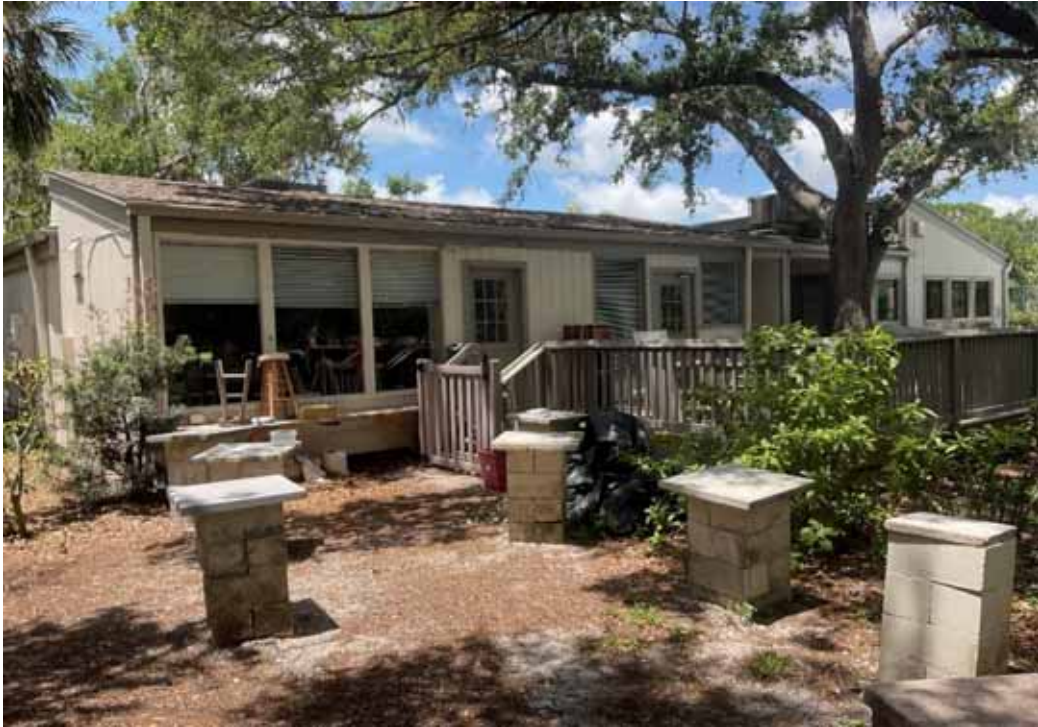
Harbor Club Recreation Building
