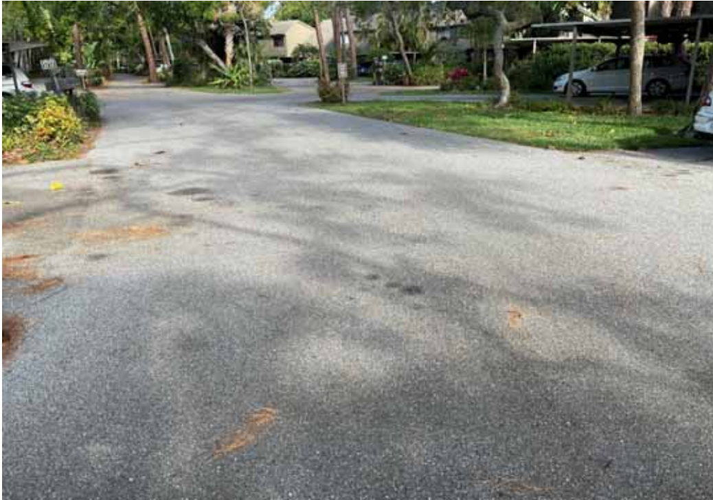
Paving - Pelican Cove Road
