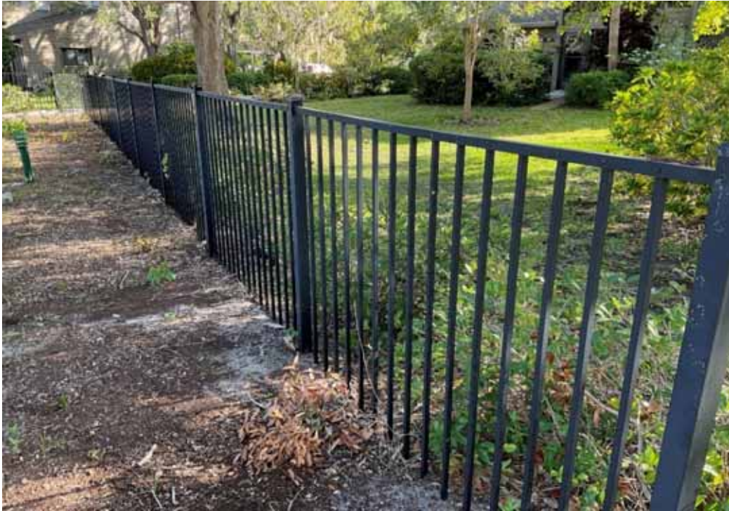
Pavilion Pool Fence
