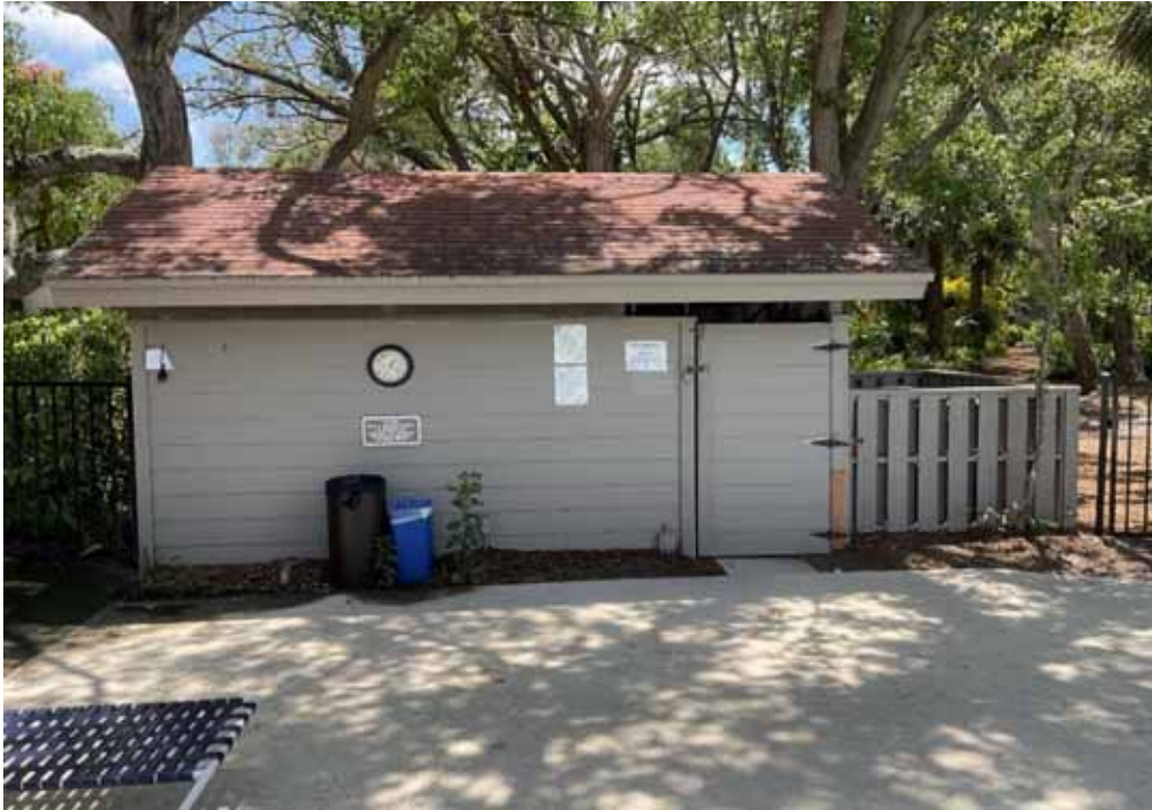
Harbor Club Pool Equipment Bldg
