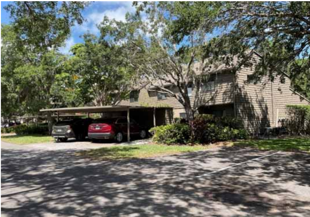
Treehouse Condo Bldg - 6 Unit
