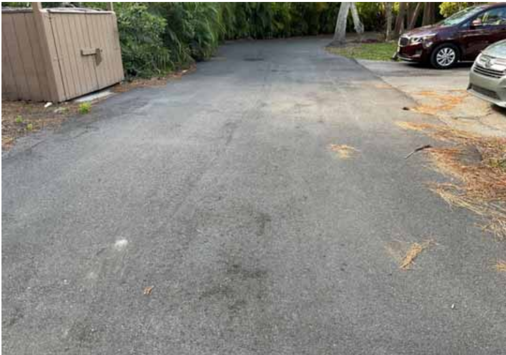
Paving - Glenhouse Drive
