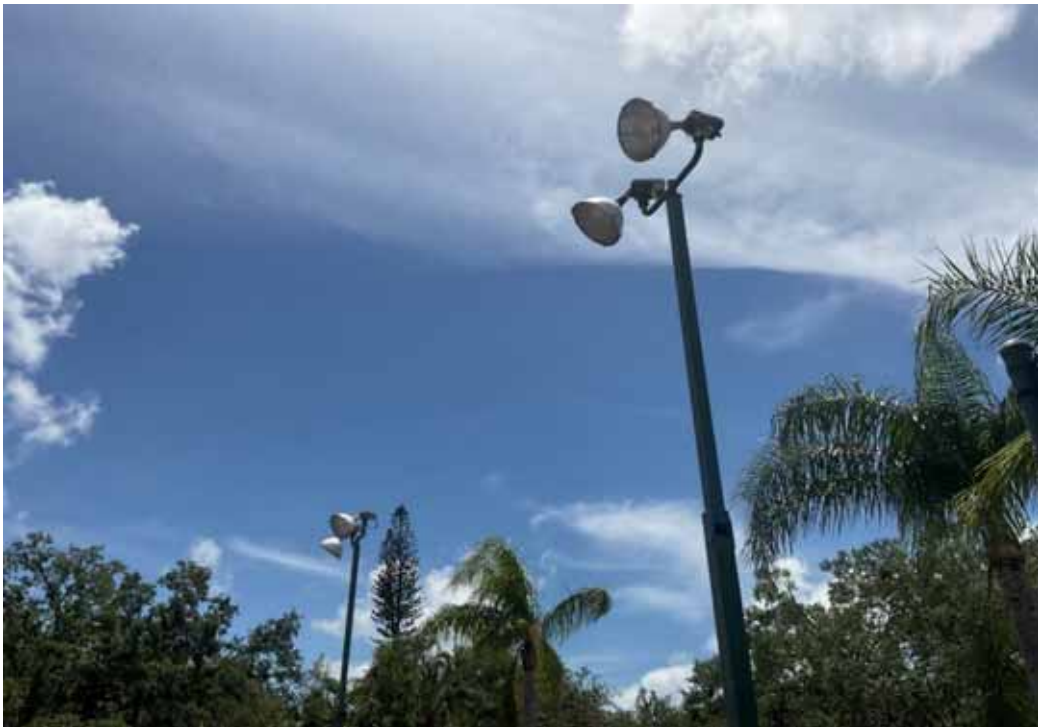
Harbor Club Tennis Court Lighting
