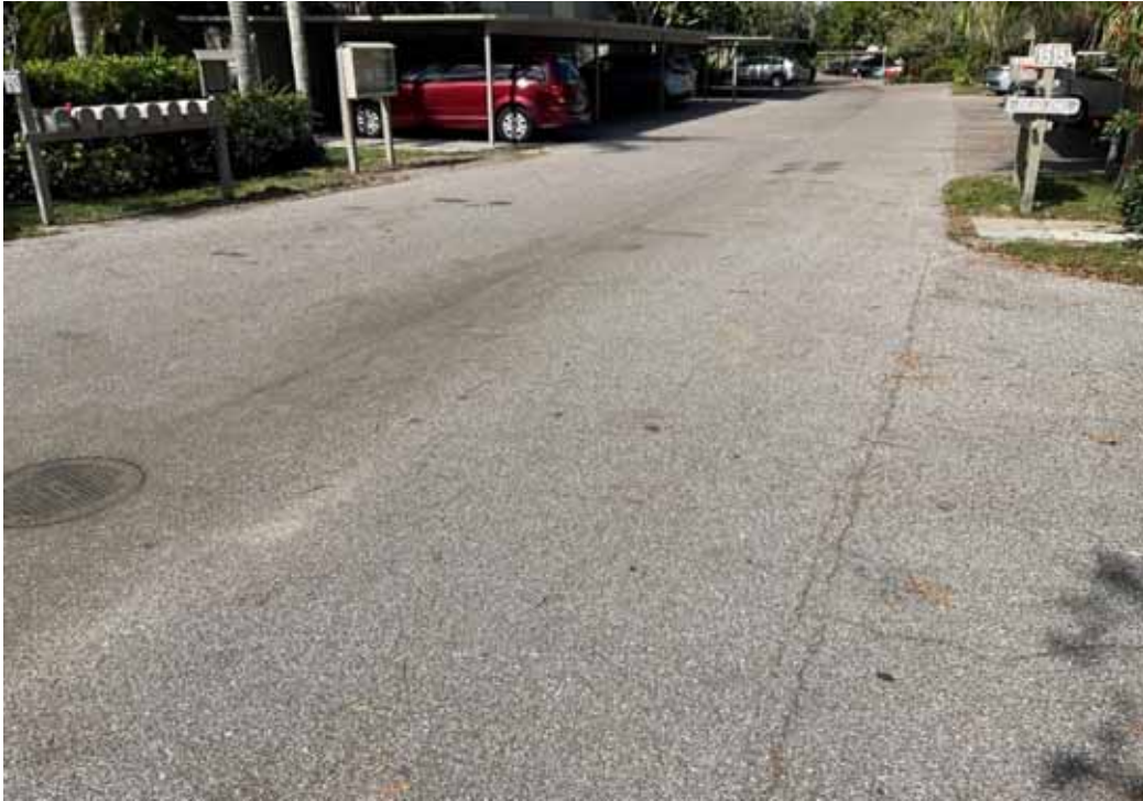
Paving - Pelican Point Drive
