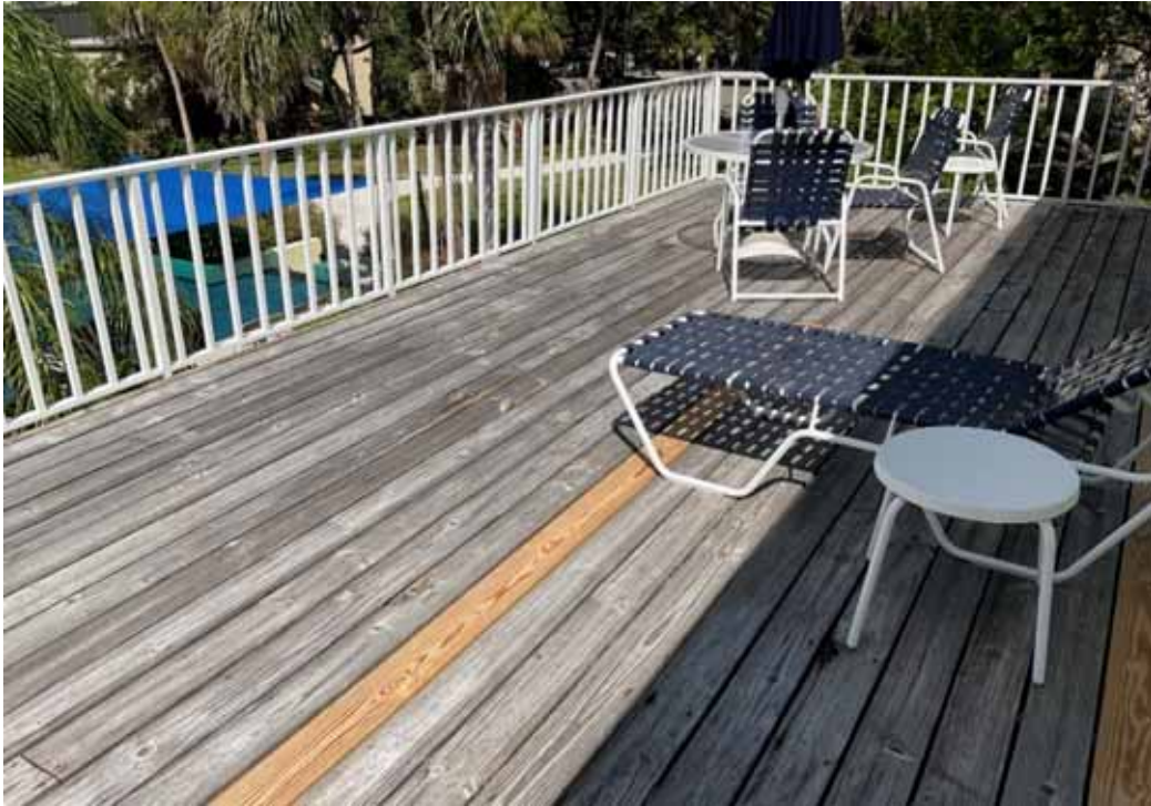
Wilbanks Bldg Second Floor Deck
