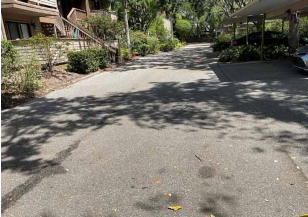
Paving - Brookhouse Circle
