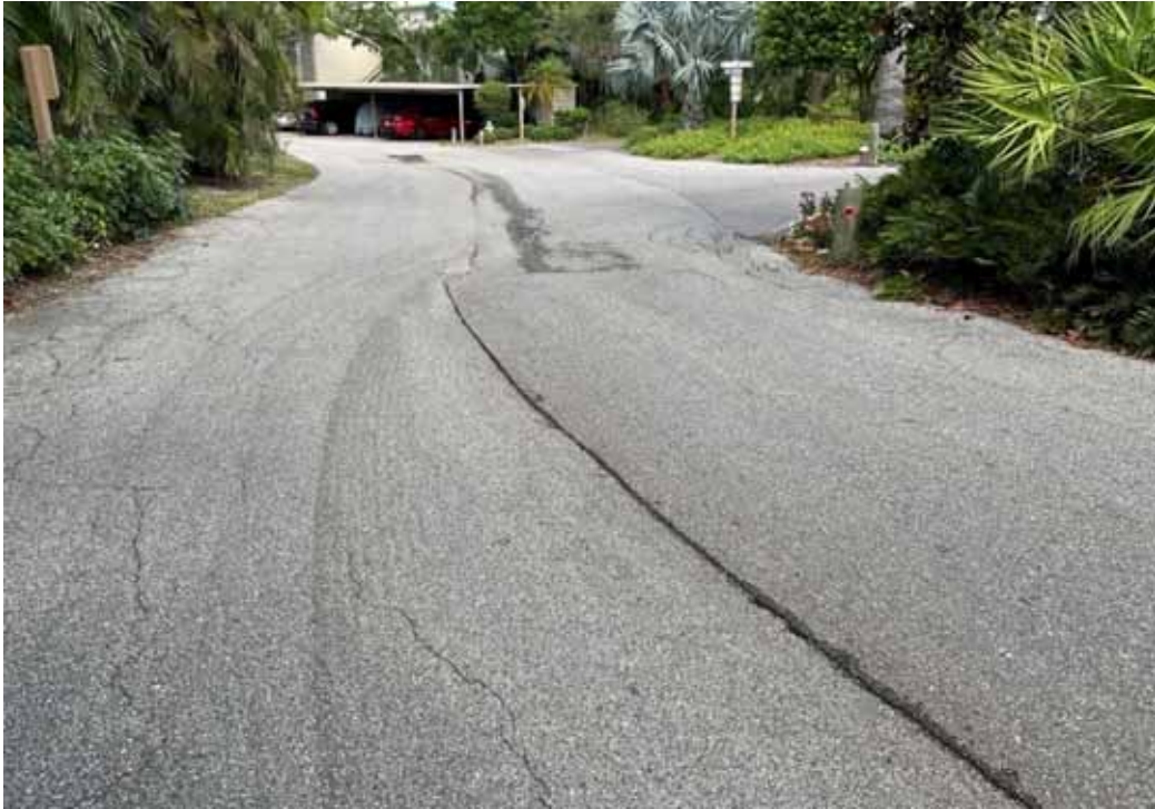
Paving - Bayhouse Point Drive
