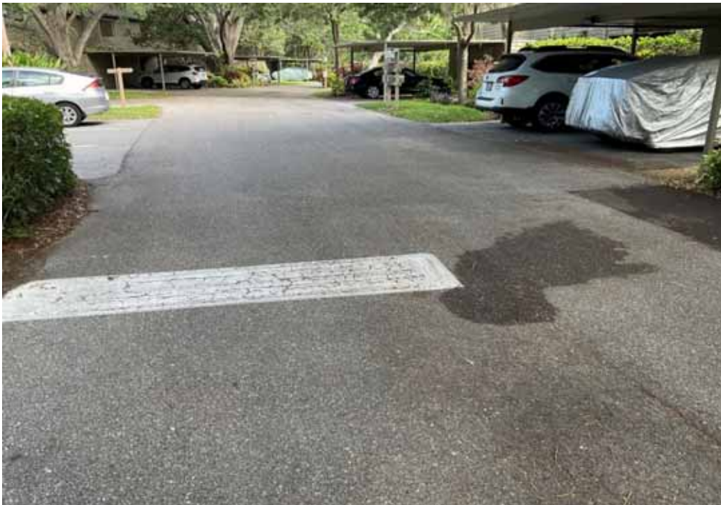
Paving - Treehouse Circle
