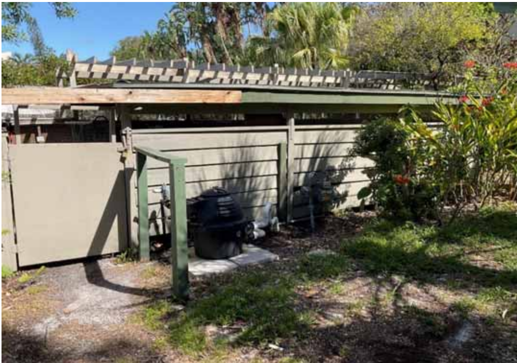
Wilbanks Pool Equipment Bldg
