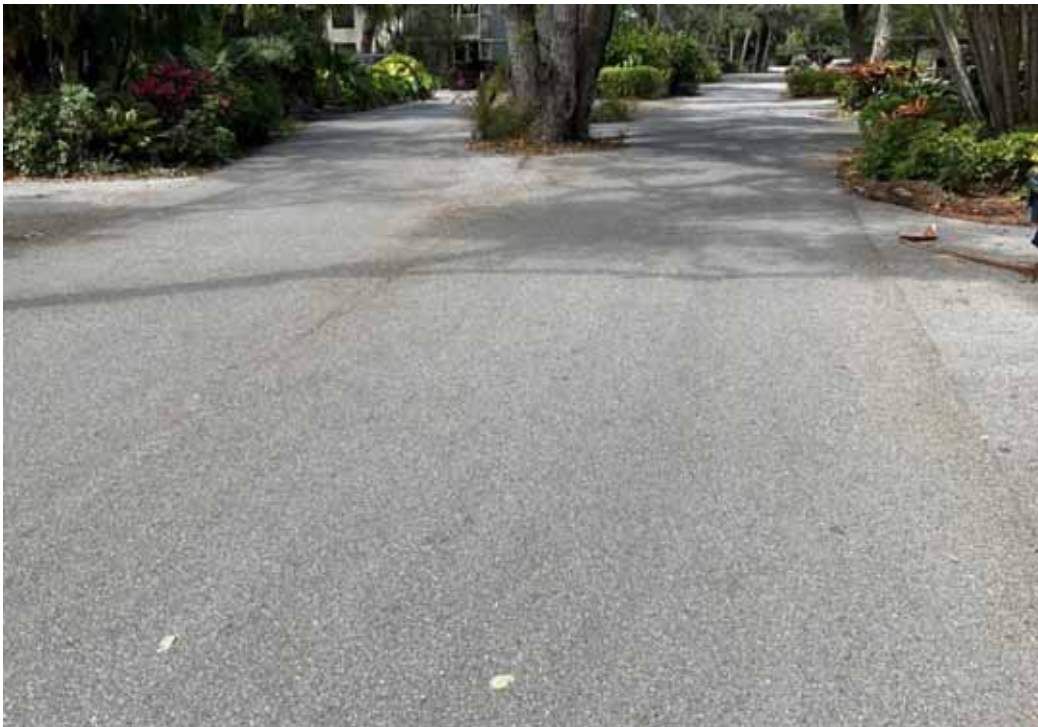
Paving - Pelican Cove Road
