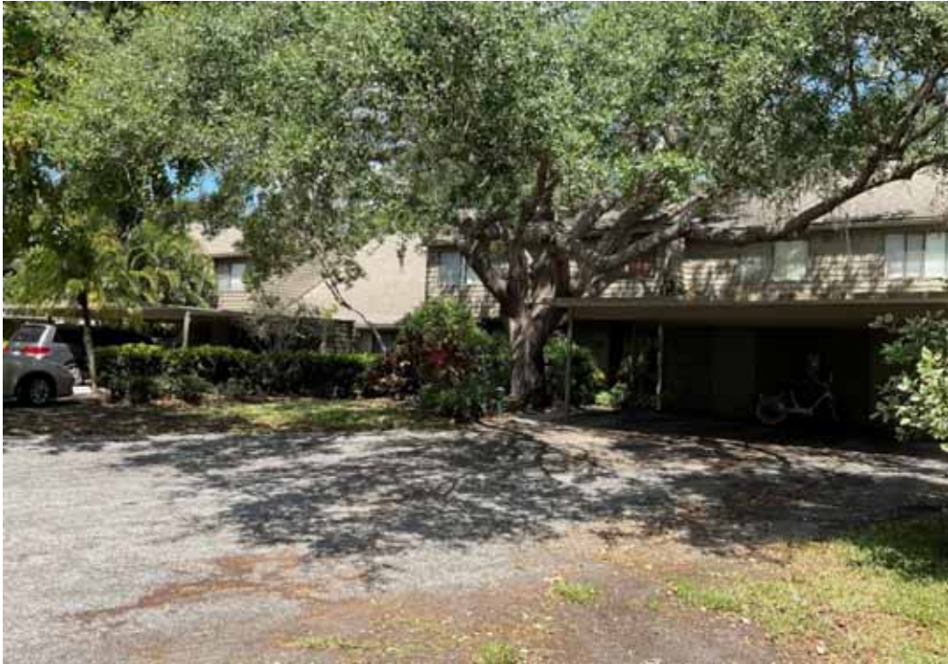
Treehouse Condo Bldg - 6 Unit
