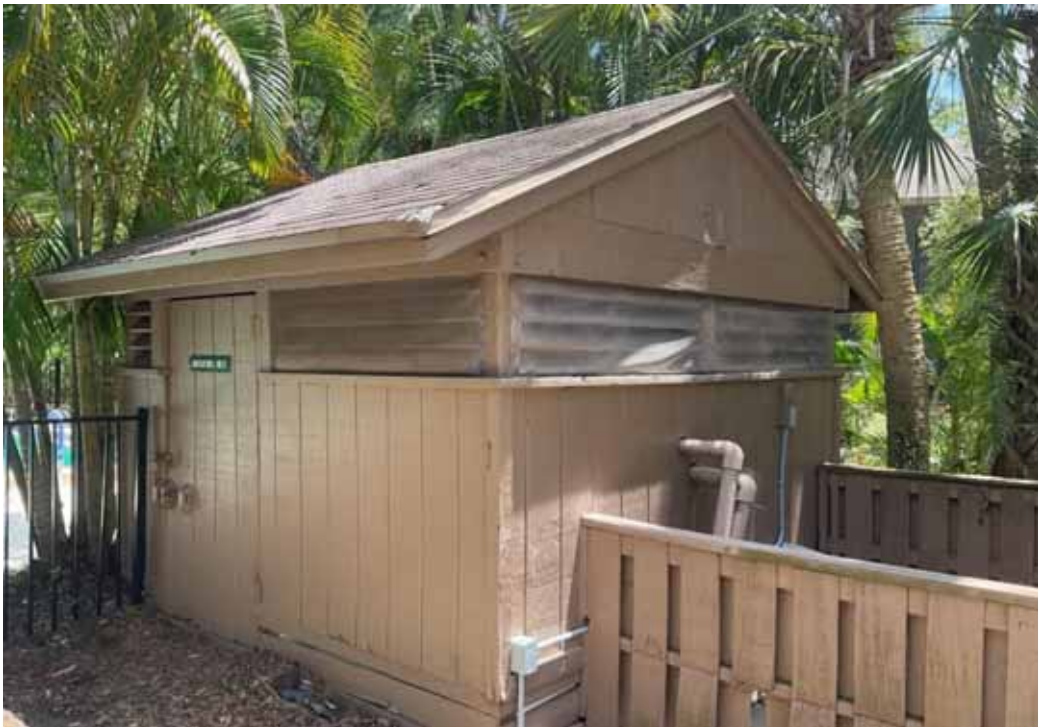
Brookhouse Pool Equipment Bldg
