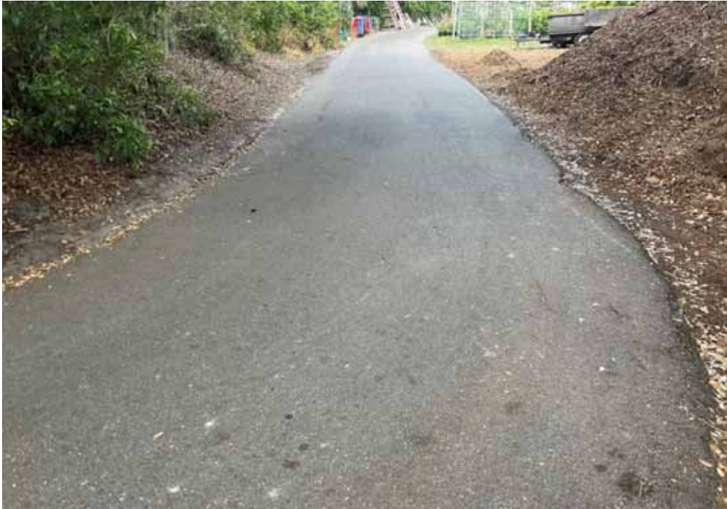
Paving - Maintenance Yard Driveway
