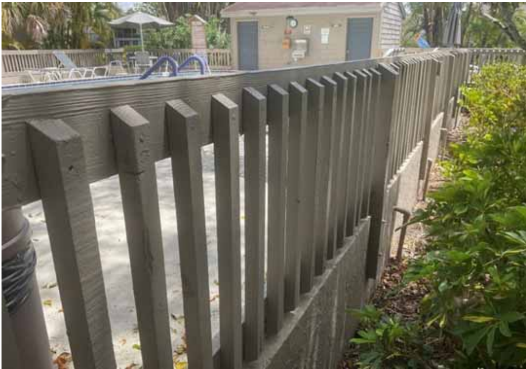
Far Harbor Pool Fence
