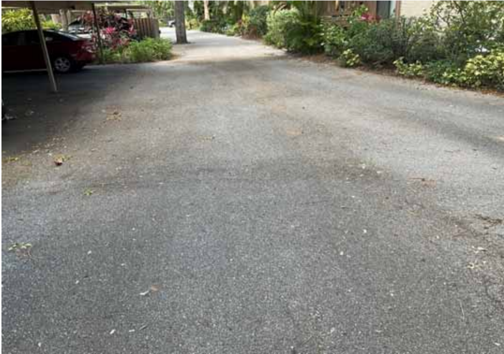
Paving - Clower Creek Drive
