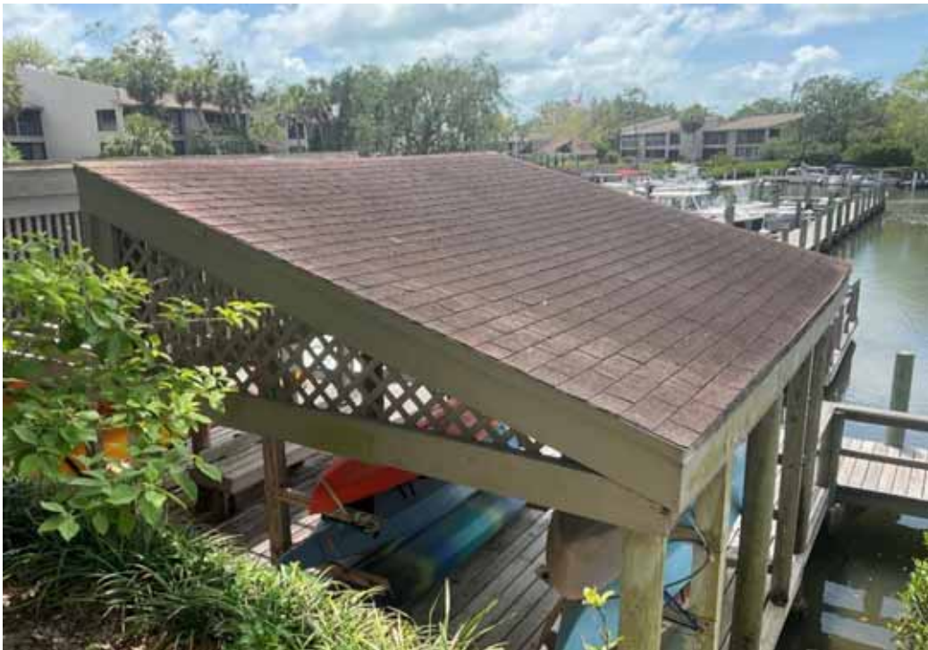
Harbor Marina Kayak Gazebo Roof
